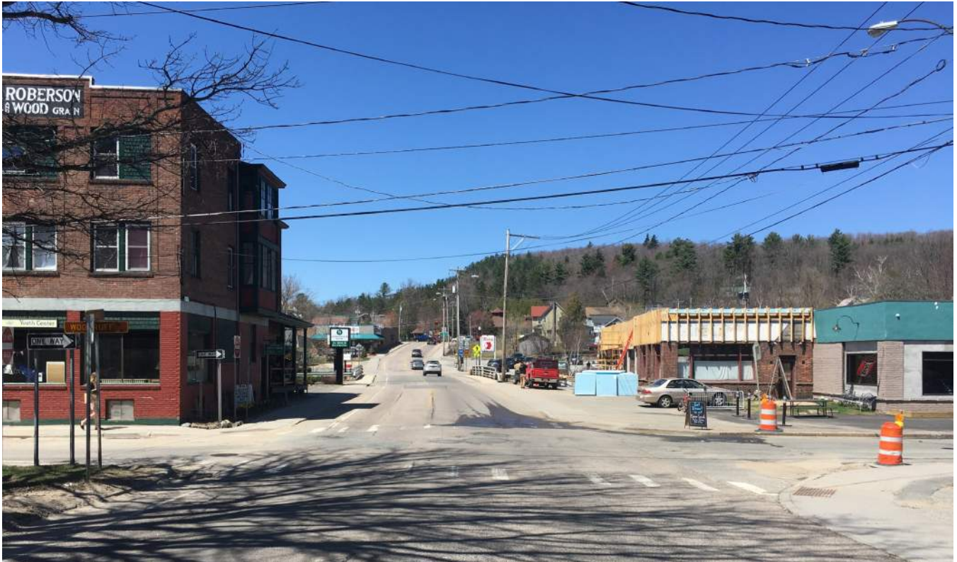
Church Street Streetscape Improvements-Existing Condition at Woodruff and Church Street
