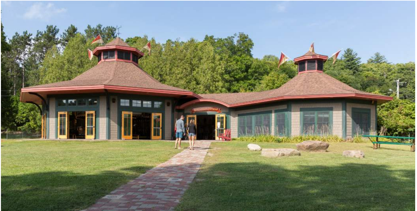
William Morris Park Improvements – Existing Conditions
