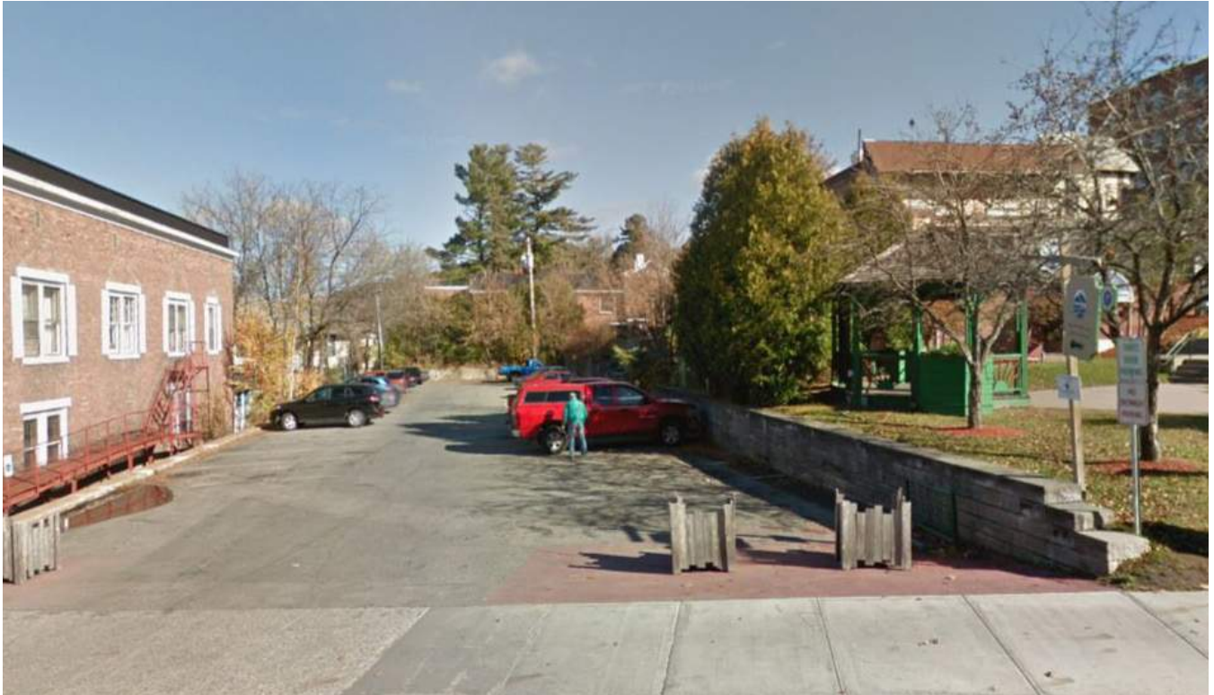
Berkeley Green Park and Streetscape Improvements- Existing Condition
