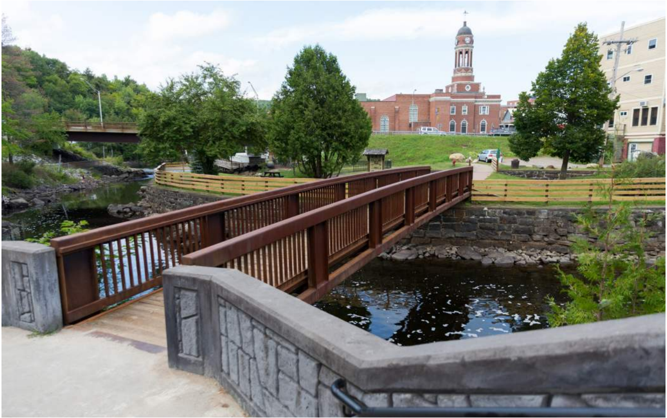
Riverwalk Completion—Existing Condition
