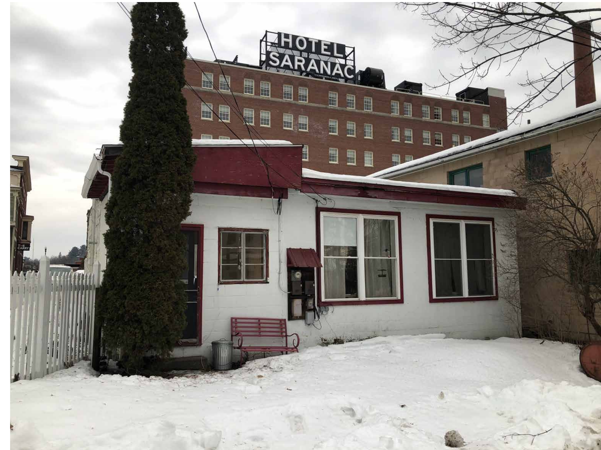
5 View of Existing South Wall
