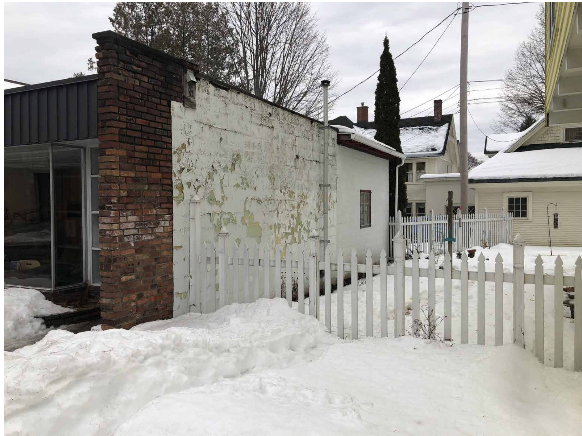
4 View of Existing West Wall
