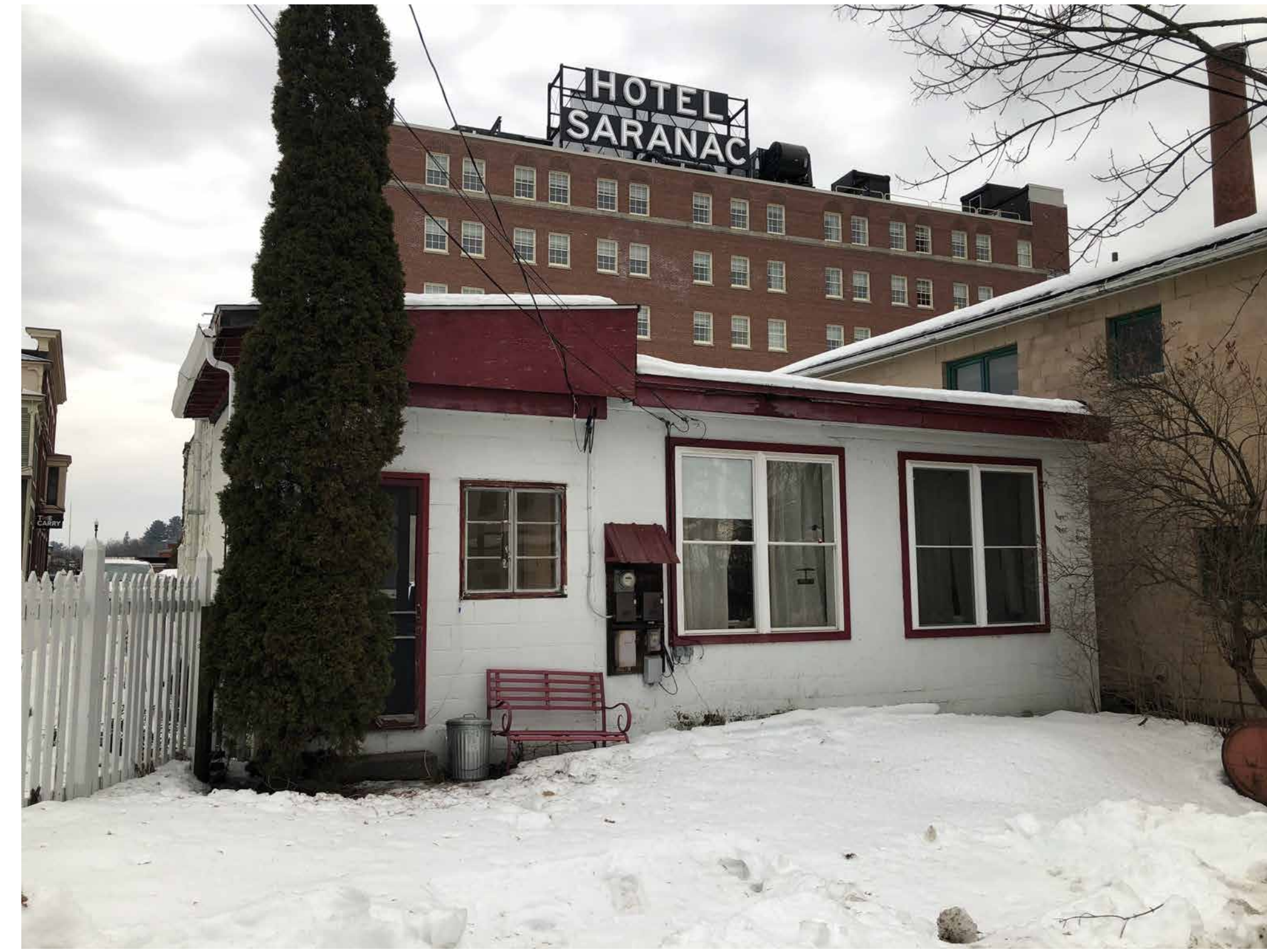
5 View of Existing South Wall
