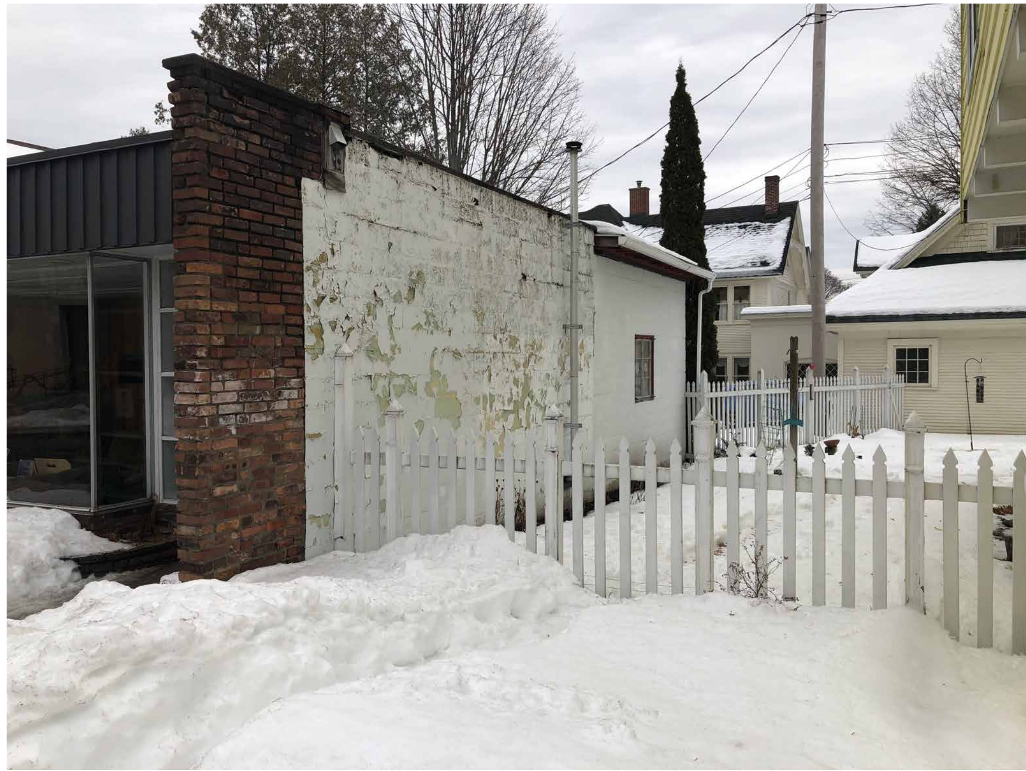
4 View of Existing West Wall
