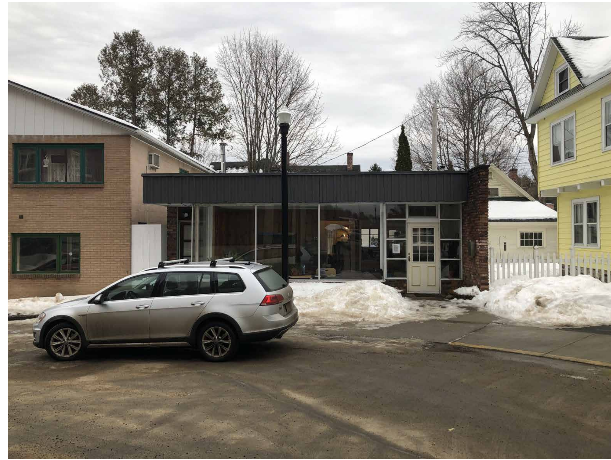
2 View from Academy Street
