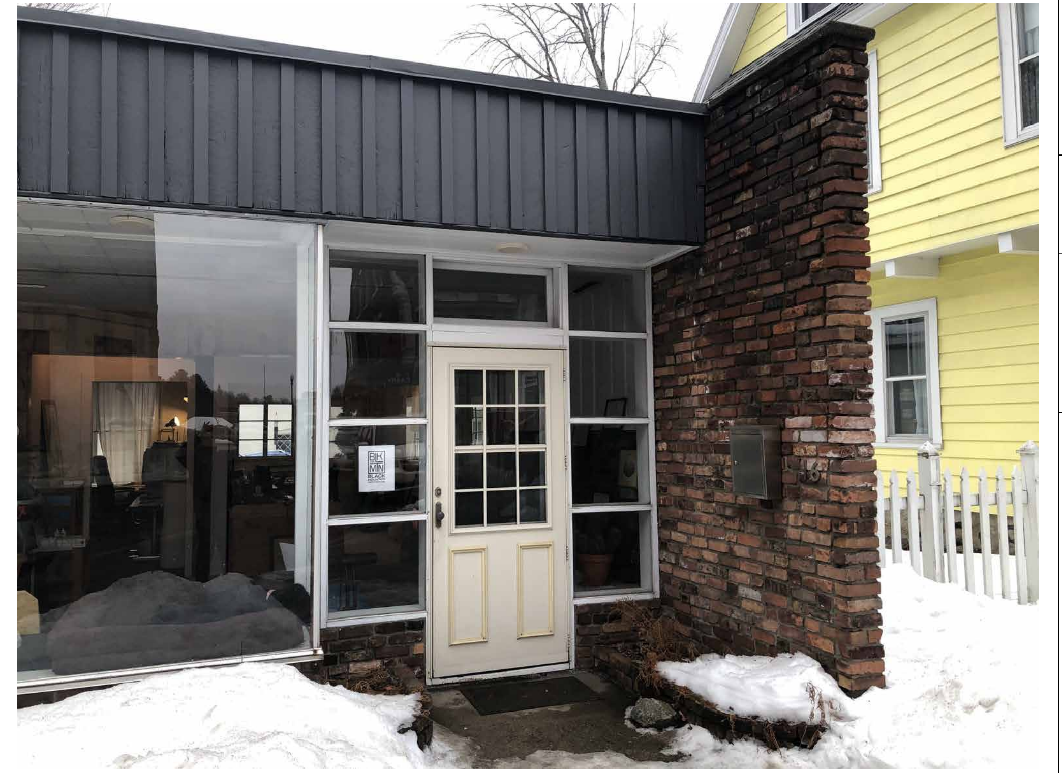
3 View of Existing Entry
