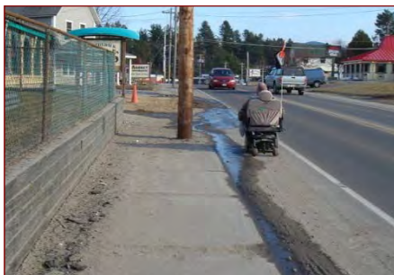
Figure 6. Narrow sidewalks are often blocked by utilities and do not provide adequate pedestrian space
