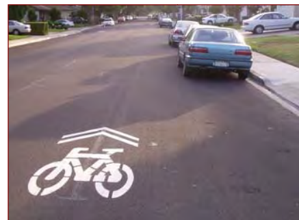
Shared lane markings can be used minor and major roadways
