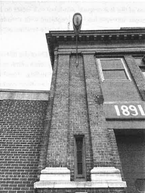
Pressed metal entablature/cornice painted red. Note stone pilaster capitals also painted red.
