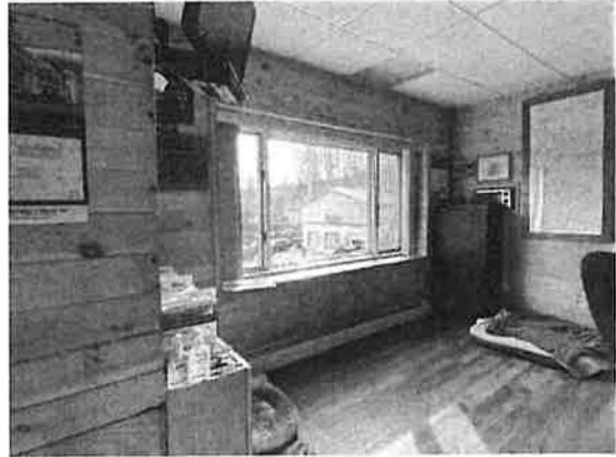
Large original window opening infilled & framed down with smaller plate glass and casement windows.
