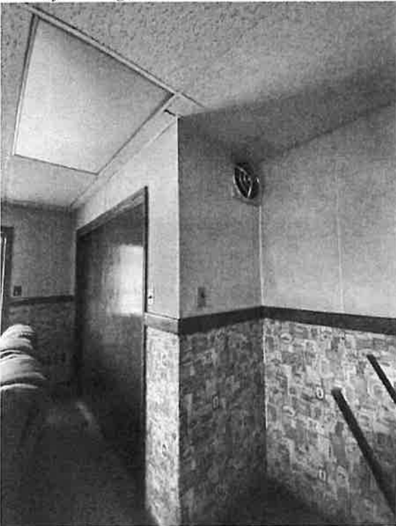
Closet built into SE corner of Kitchen is modern with hollow core sliding doors. Masonite paneling covered with wallpaper.
