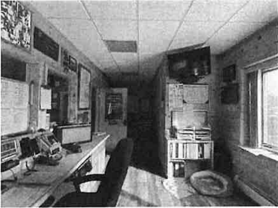
Subdivided Dispatch Room finished all in knotty pine horiz. boards with acoustical tiled ceiling.
