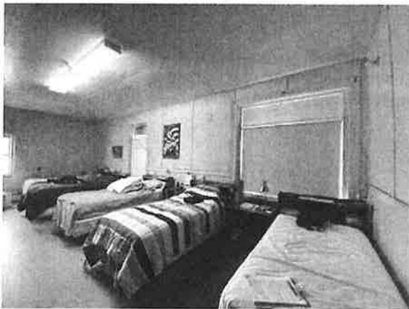
South and east walls of Bunk Room show how original window openings have been retained but have modern replacement units.
