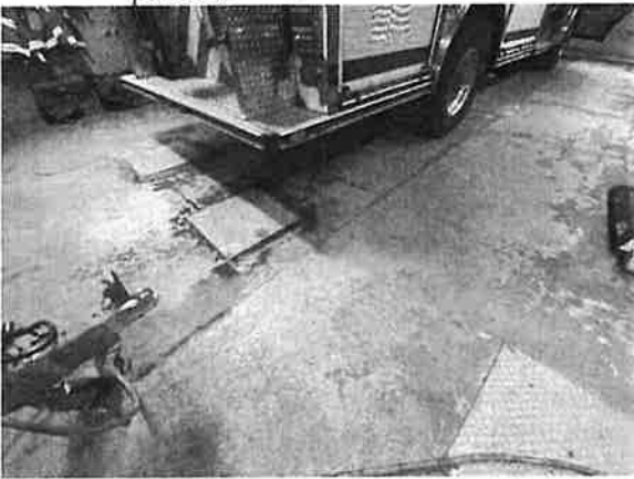
Detail view of patched concrete floor of garage bay.
