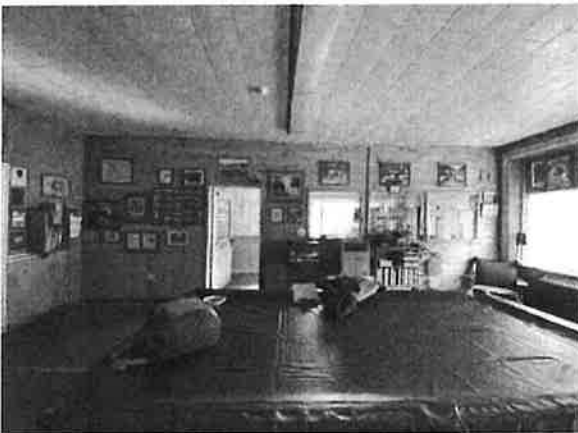
Modern south partition wall of Day Room constructed of knotty pine boards & fixed windows – out of character of orig. finishes.
