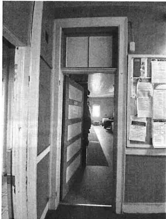
Doorway to bunk room retains original trim surround, transom (glass painted) and paneled door.
