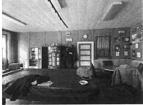
North wall of 2 nd floor Day Room showing paneled wall sheets with battens & original 5-paneled door to closet.
