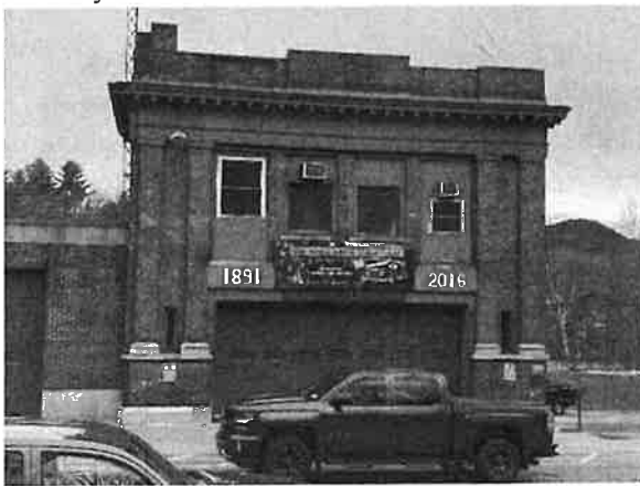
Front elevation with altered 2 nd floor window/door openings and missing balcony.
