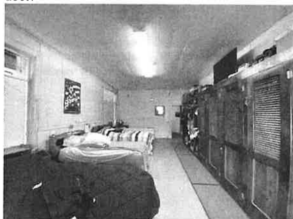
Historic wall, ceiling and floor finishes covered with layers of vinyl tile, acoustical tile and Masonite sheet paneling.
