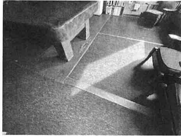
Linoleum sheet flooring pieced together with stainless steel threshold strips. Likely over orig. wood flooring.
