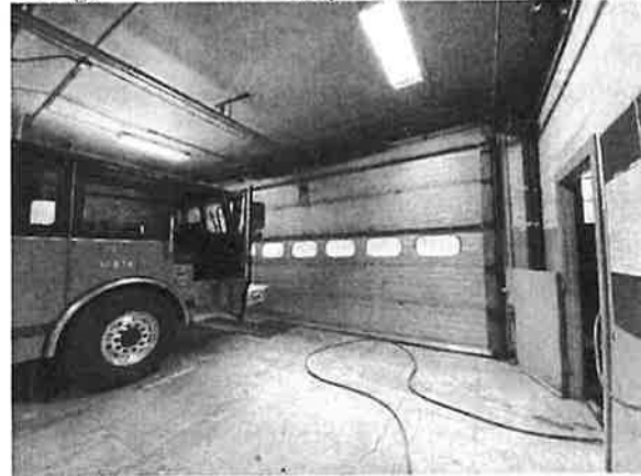
Detail view of modern overhead door on front wall.
