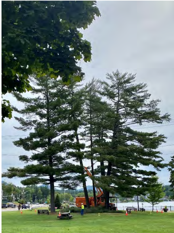
Tree removal at Riverside Park
