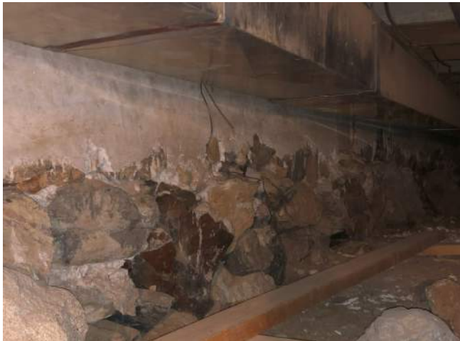
Photo #1 – Stone Rubble & Concrete Foundation
