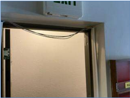
Exhibit 15 - Exposed cables above doorway.
