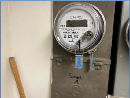
Exhibit 2 – Service A meter with error message E01
