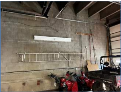
Exhibit 8 – Fluorescent linear utility light – lower level
