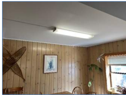
Exhibit 11 – Fluorescent surface light fixture
