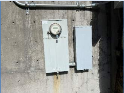
Exhibit 2 – Town Office and Marshall Building electrical service meter and service disconnect
