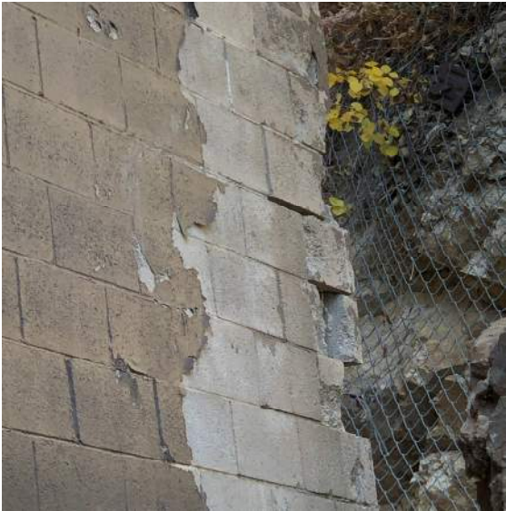
Photo #3 – Damaged CMU Walls
