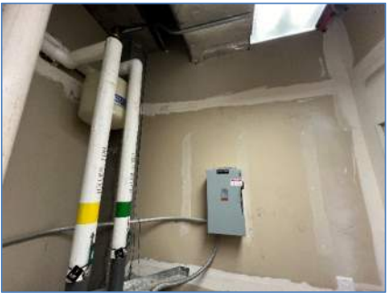
Exhibit 7 – Mechanical duct above the boiler disconnect
