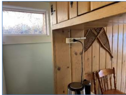
Exhibit 9 – Existing wiring devices and surface raceway
