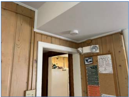
Exhibit 12 –Emergency bug eye and toggle switch
