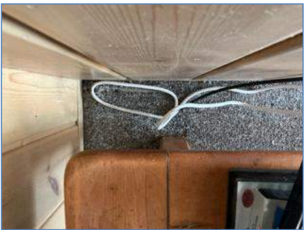
Exhibit 15 – Coax cable punched through floor
