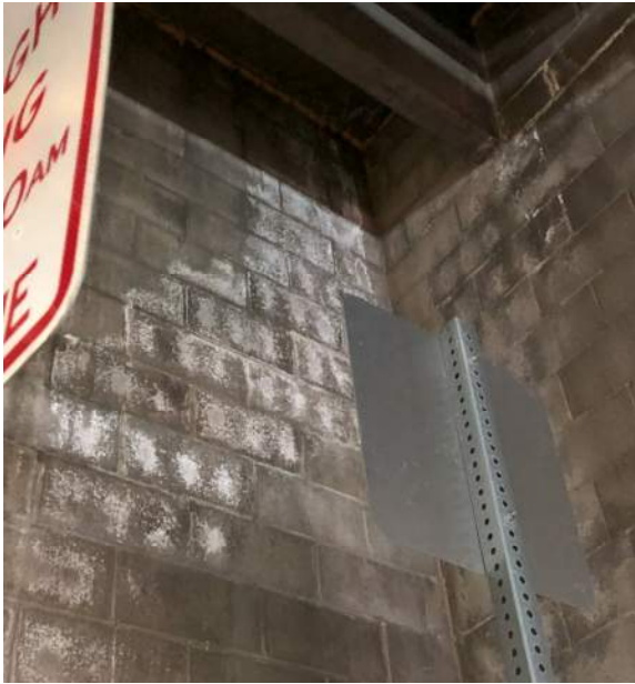
Photo #4 – Moisture Infiltration in CMU Walls
