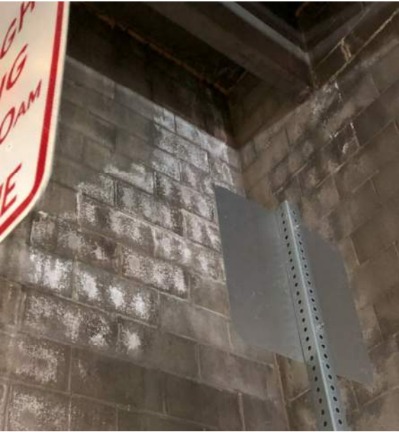
Photo #4 – Moisture Infiltration in CMU Walls
