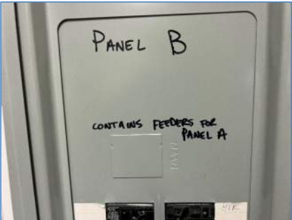
Exhibit 4 – Panelboard B note for panel A feeder
