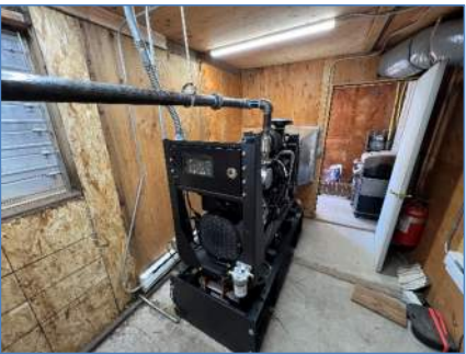
Exhibit 6 – Standby generator in the Marshall Building
