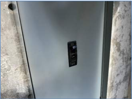
Exhibit 4 – Town Office and Marshall Building electrical service main service disconnect – 150A
