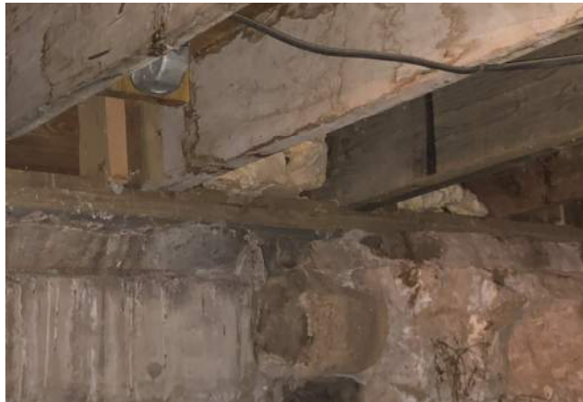
Photo #2 – Floor Joists Resting on Foundation
