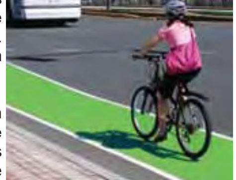
Example of Epoxy Bike Coating on Asphalt
