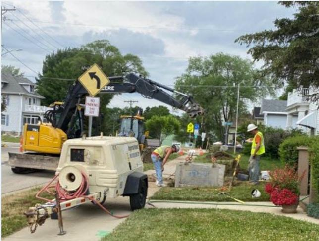
A Stoughton crew replaces a lead service line. The city successfully used directional drilling for most LSL replacements and only dug open trenches in situations where other methods were not feasible.
