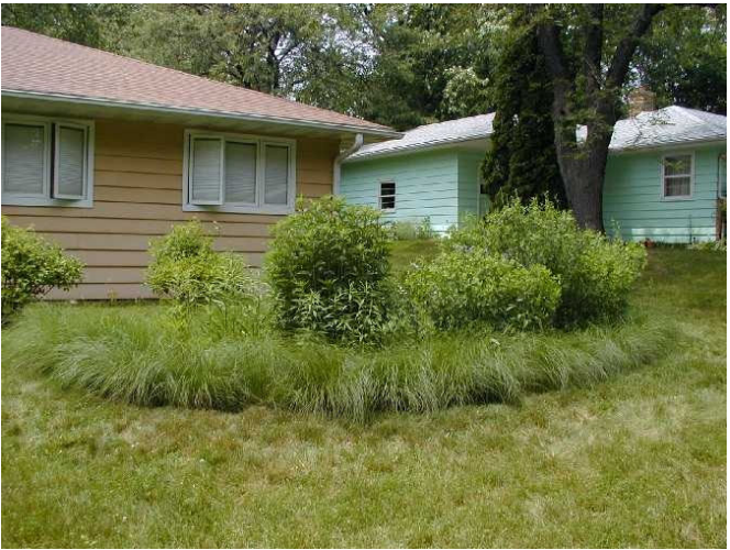
A front yard rain garden next to roof downspout. (Source: UW-Extension)
