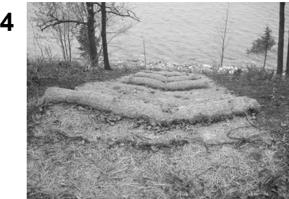
Erosion matting is used on steep slopes to shield bare soils and prevent new plantings from washing away during rain storms.
