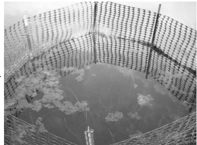
A variety of bulrushes are planted in the water in front of the recently-installed rock. At maturity, they will poke above the water surface. Temporary snow fencing protects the shallow-water plantings from waves and animal grazing.
