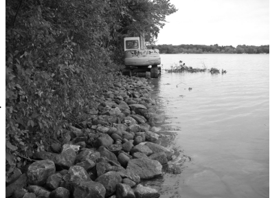
Glacial boulders are anchored into the 870-ft. shoreline, providing long-term erosion control on this exposed peninsula.
