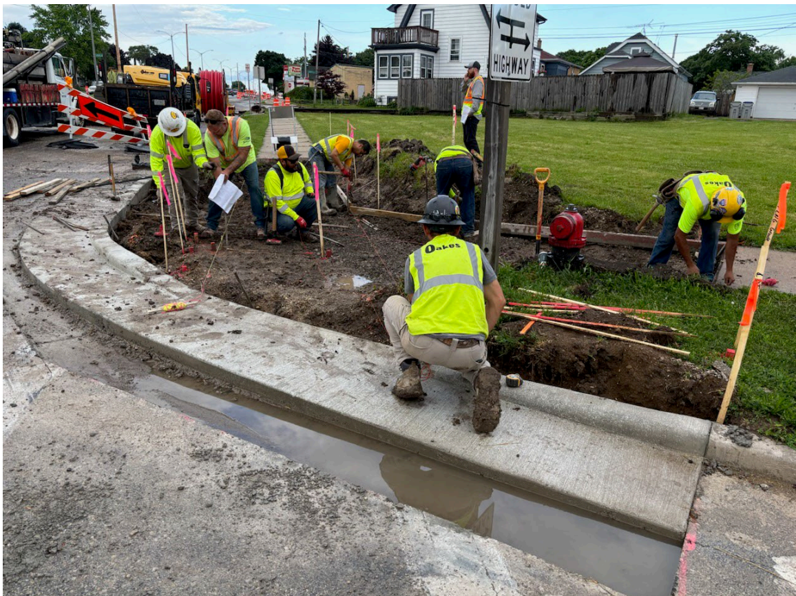
Setting forms for concrete sidewalk
