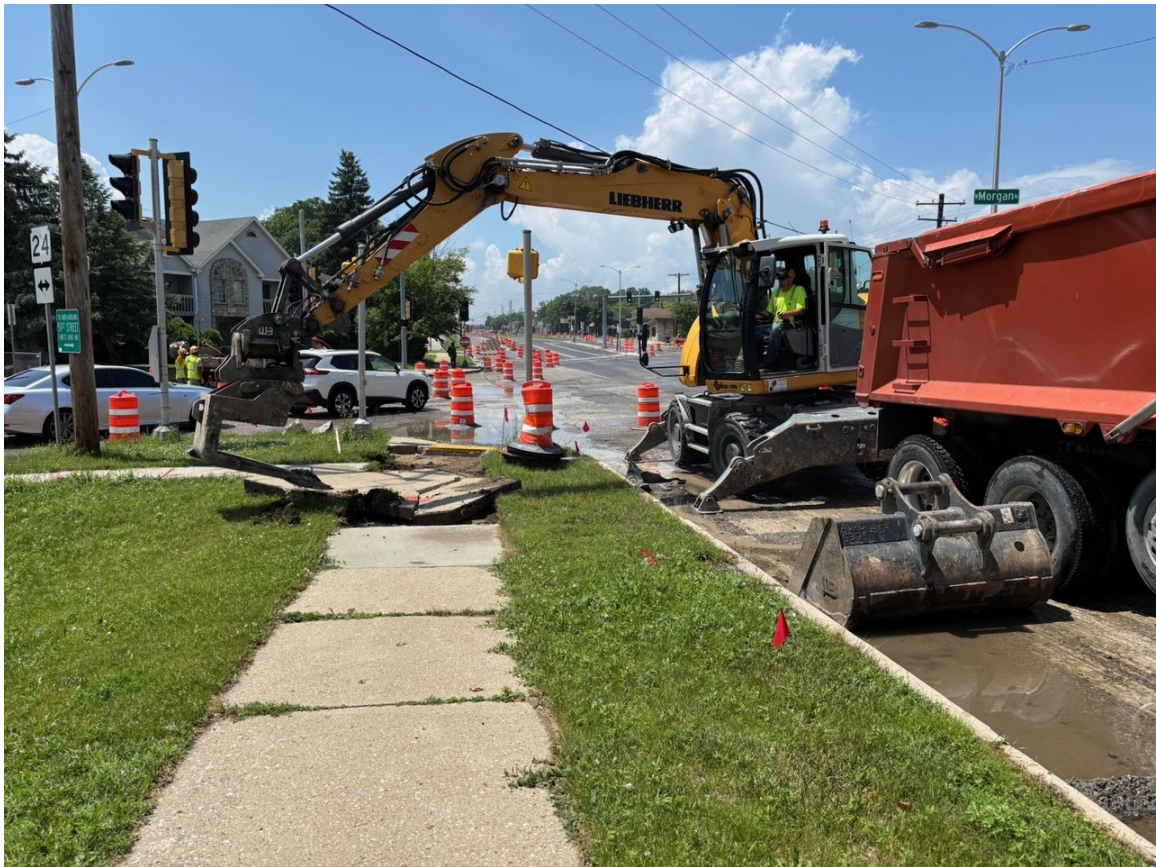
Removing Curb and Sidewalk at Morgan Ave & Forest Home
