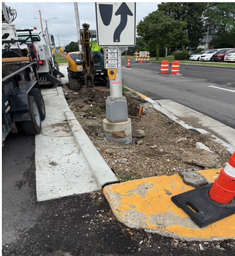
Installing a traffic signal pull box in the median island
