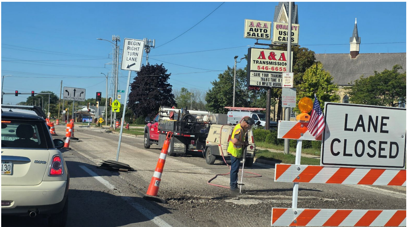
Cleaning pavement joints in preparation for repairs
