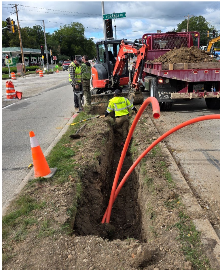
Installing conduit in the median for traffic signal interconnect
