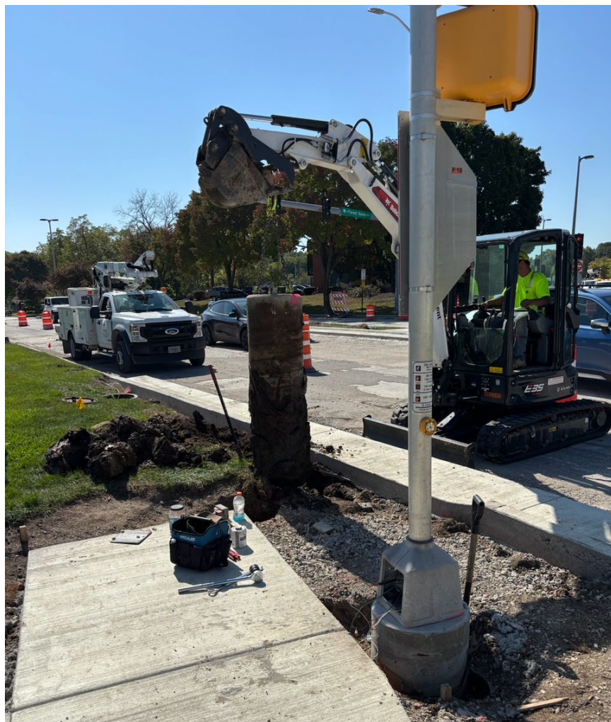
Removing old traffic signal bases
