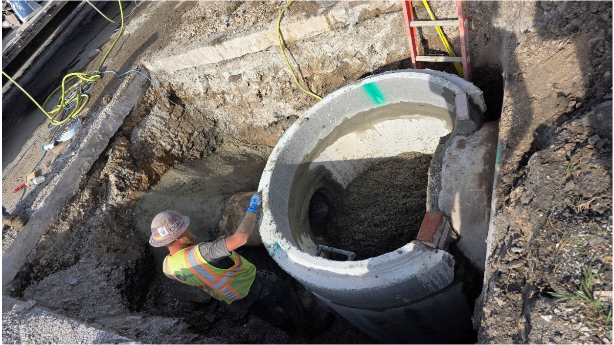
Installing a storm sewer inlet
