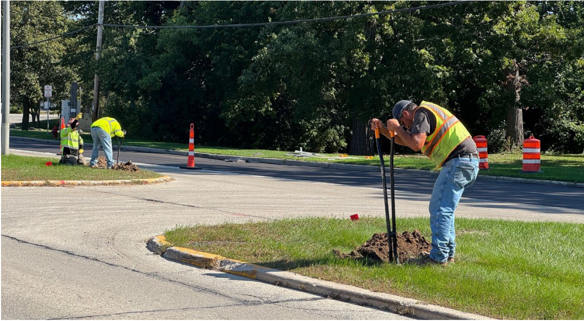
Removing old traffic signal bases
