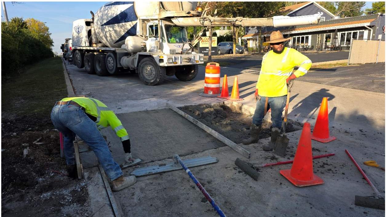
Placing base patch for in pavement for traffic signal loop installation
