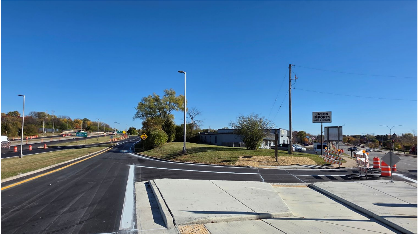
Application of epoxy pavement markings Layton Ave ramp
