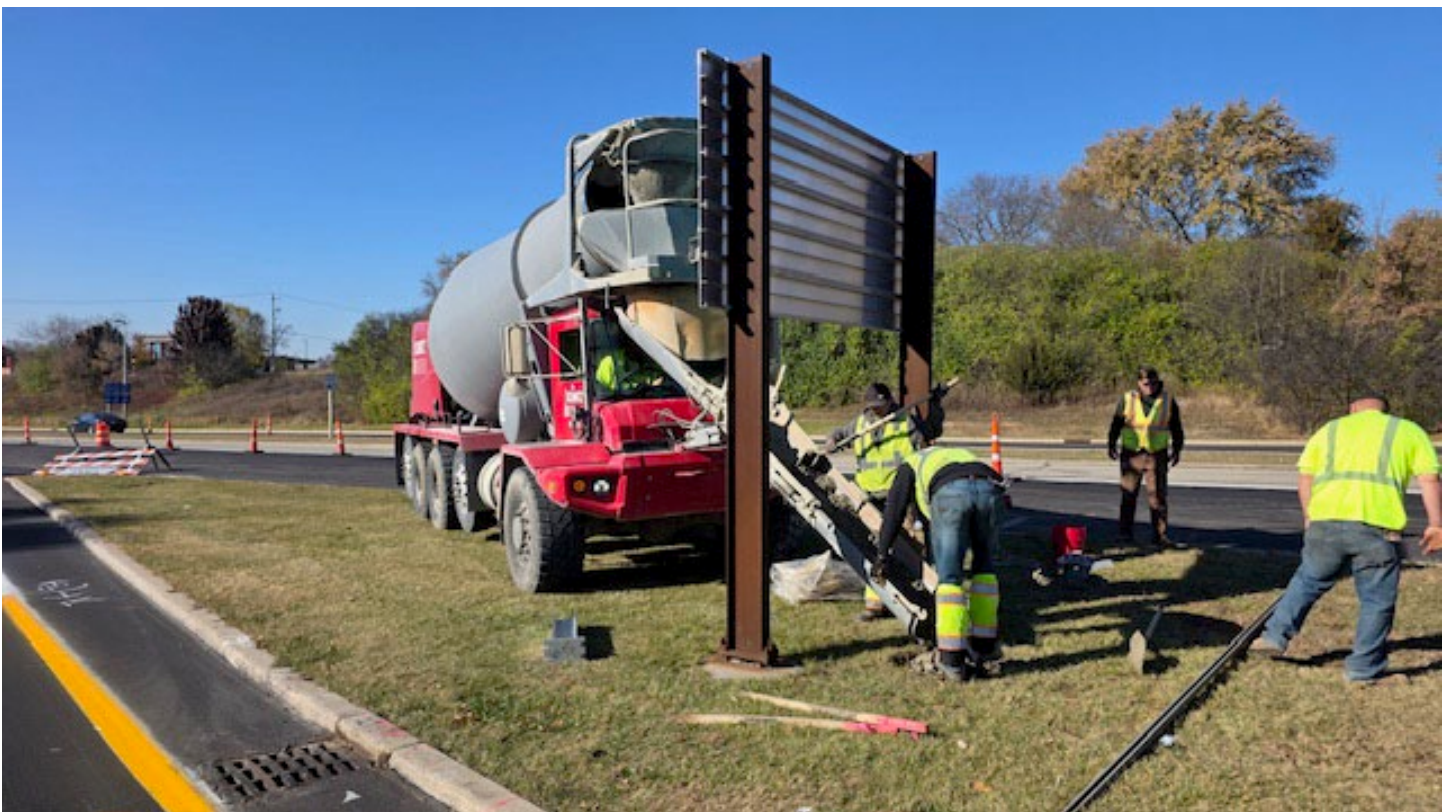
Placing concrete for a new Type I sign bases
