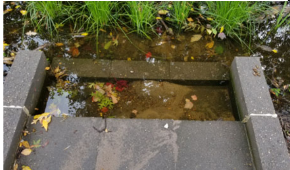
Custom Concrete Forebays
