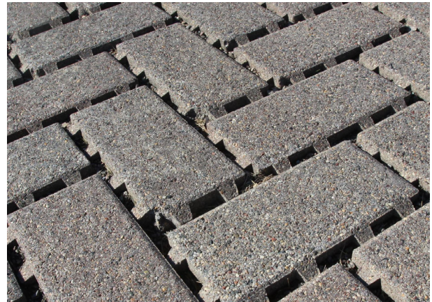
Figure 19: Permeable Concrete Pavers
