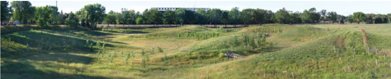
Figure 21: Infiltration Basin doubling as recreational space
