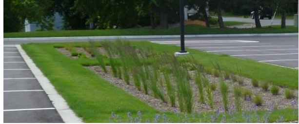
Figure 15: Vegetated Filter Strip
