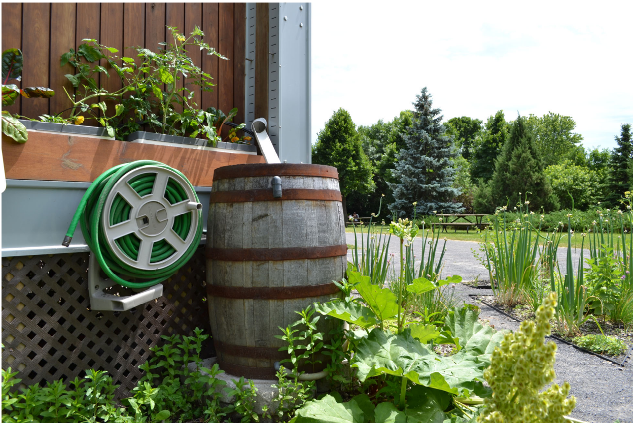
Figure 26: Rain barrel for harvesting roof runoff
