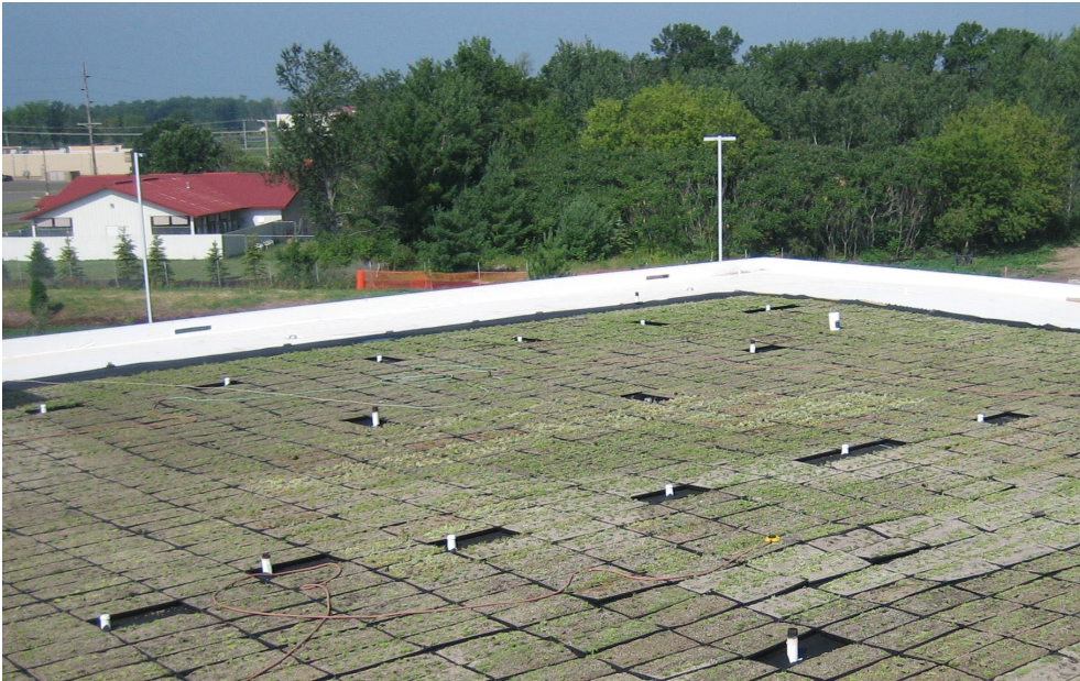
Figure 27: Green Roof on Amery Regional Hospital (EOR)
