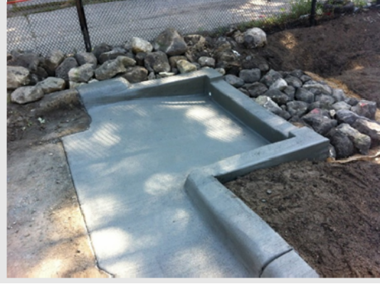
Custom Concrete Forebays
