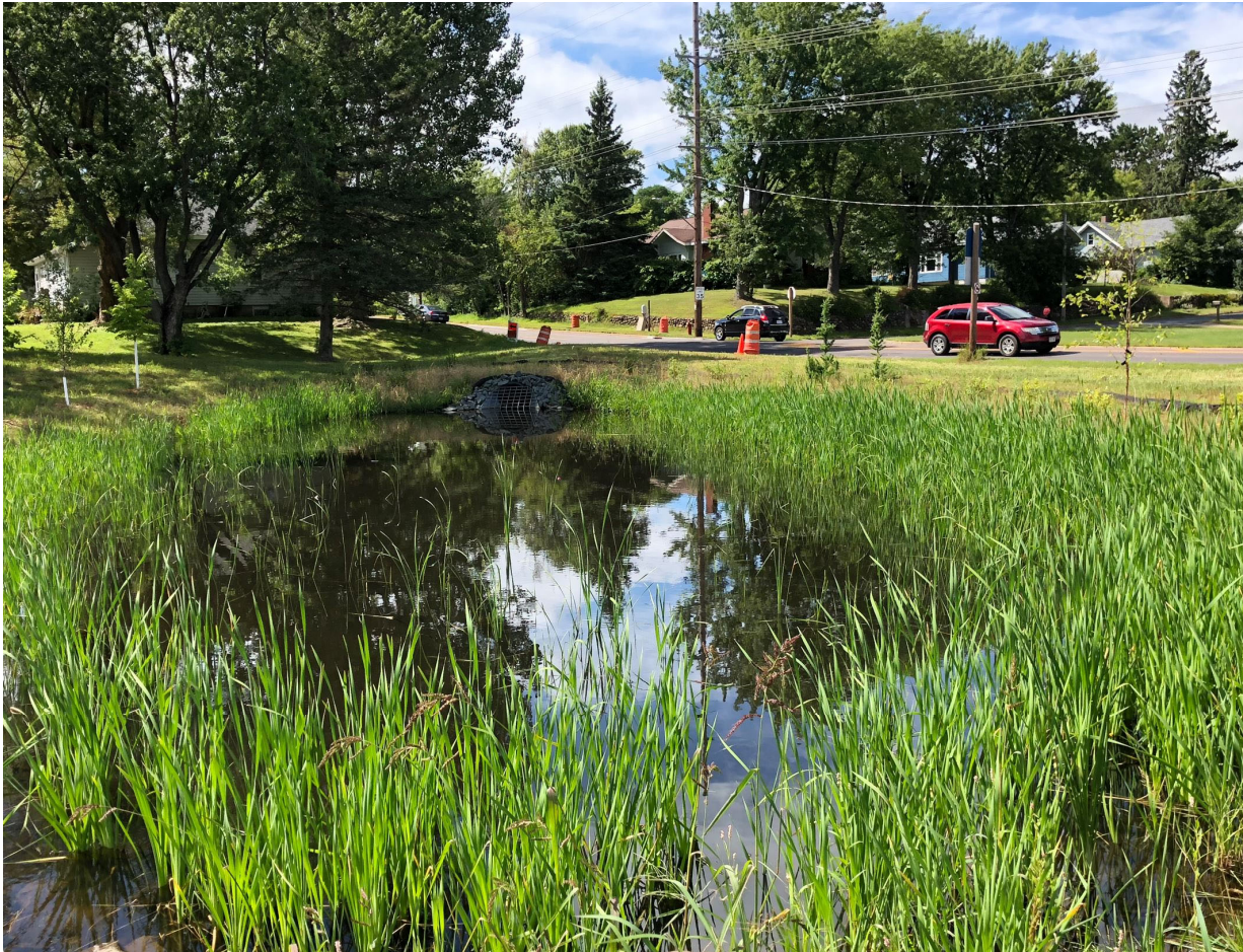
Figure 28: Stormwater Wetland in Cumberland (EOR)
