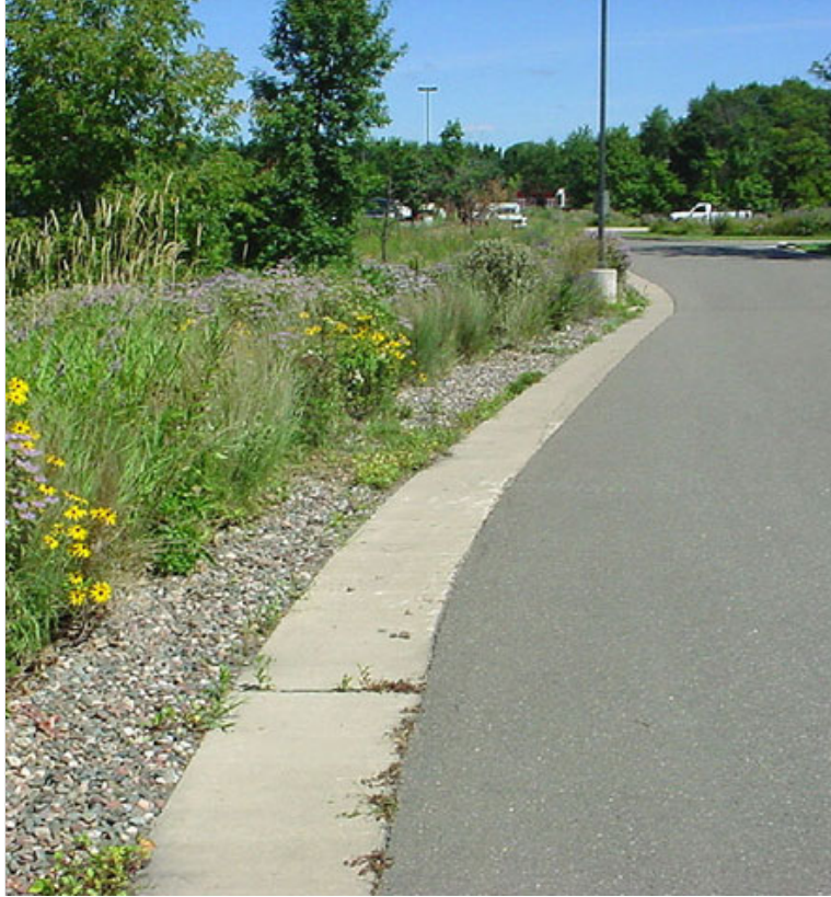
Figure 22: Infiltration Trench (MPCA)
