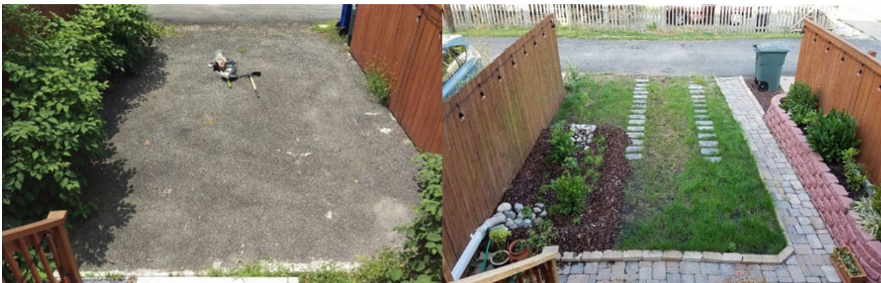
Figure 9: Impervious cover removal in backyard ( https://www.riversmarthomes.org/isr )
