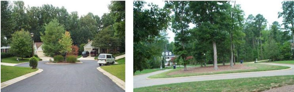
Figure 10: Trees and Vegetation Planted in the Landscaped Island of a Cul-de-sac (left) and a Loop Road (right) (Minnesota Pollution Control Agency 2013)
