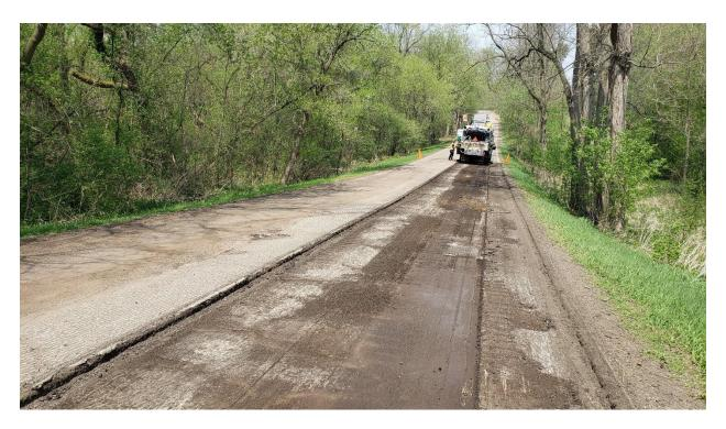
The base stone is then recompacted and 4" of HMA binder is placed to match the existing pavement elevation ready for resurfacing as shown here. This work was performed with a special mobilization the day before to allow for the binder patching to cool and cure overnight.
