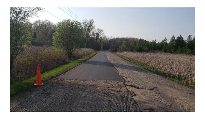
Unfortunately, thre was another area that didn't look to distressed until the loaded trucks drove over it which caused an emergency repair to be performed in order to keep paving as shown here.
