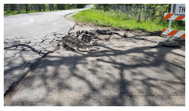
It was found that there was only 3" of aggregate base below this pavement and then 3' of extremely soft silty clay. This excavation was performed by the Town DPW forces. Stark Pavement assisted with placing and compacting the base stone and installation of a thick binder base patch to bridge the soft material. To make things more difficult, there was a high-pressure gas main running directly in the middle of the patch.
