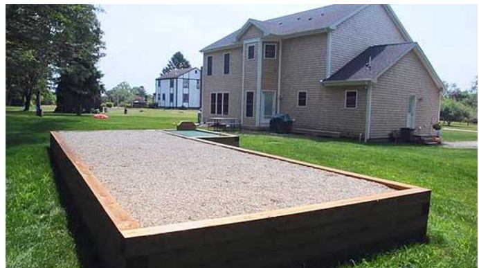
Recirculating sand filter system. Images courtesy (from top): USEPA; AJFoss.com
