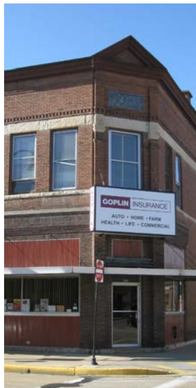
NOT PERMITTED This wall sign covers up the second-story window sill and the first floor cornice and it extends beyond the corners of the facade walls. A projecting sign between the windows or a sign mounted on the canopy would be preferred in this case.
