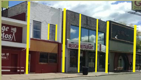
APPROPRIATE Vertically-proportioned buildings with articulation of structural bays and tall windows.
