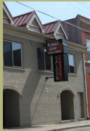
NOT PERMITTED The projecting sign is placed in front of a window while an alternative location between the windows is available.
