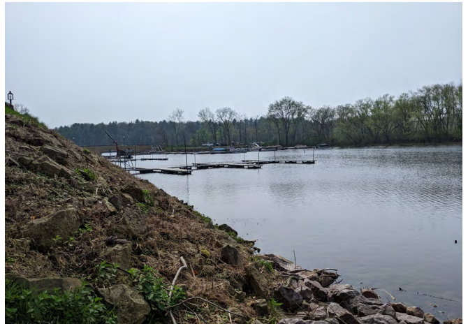
Boat Launch Ramp (Indiana Avenue Boat Launch) Municipal Docks (Illinois Avenue Boat Docks)
