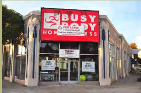
NOT PERMITTED This wall sign obscures the existing architectural features, including part of the windows, and is out of proportion to the building mass.
