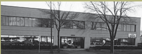
NOT PERMITTED Wide building with no vertical expressions to break up the facade.
