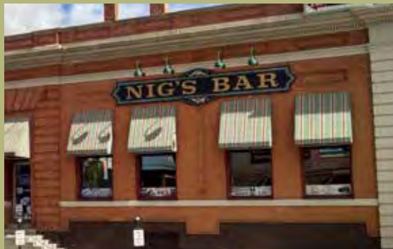
APPROPRIATE This sign is placed well within the existing architectural features (centered on the brick inlays and above the window/ awnings , but below a cornice line).
