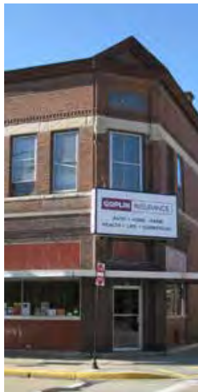
NOT PERMITTED This wall sign covers up the second-story window sill and the first floor cornice and it extends beyond the corners of the facade walls. A projecting sign between the windows or a sign mounted on the canopy would be preferred in this case.
