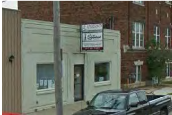
NOT RECOMMENDED This projecting sign reads well from the sidewalk, but less so from the roadway due to its orientation and the small text.
