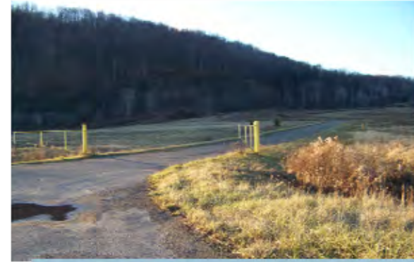
SITE ENTRANCE AND ACCESS ROAD
