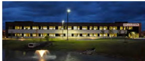
DRESSER RAND IS A MAJOR EMPLOYER IN THE REGION AND IS LOCATED IN THE STUDY AREA. (SOURCE: WWW.BUILDWELLIVER.COM)
