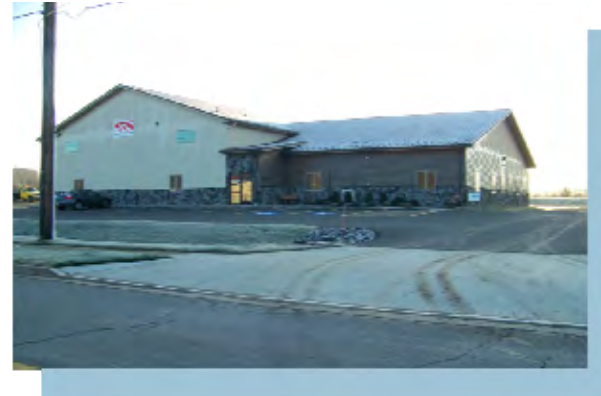
VIEW OF SITE FROM FRANKLIN STREET
