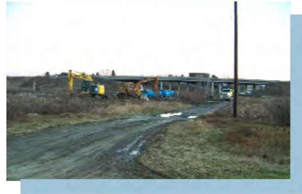
VIEW OF ONGOING SITE REDEVELOPMENT
