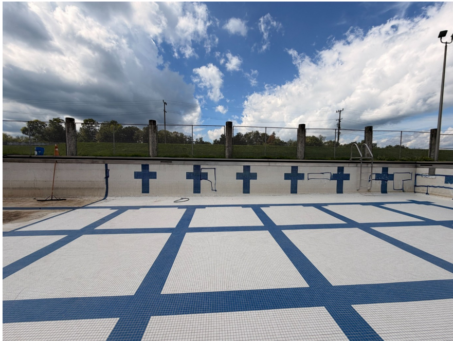
Photo 4 Opposite wall overview. Existing tile finishes, marked wall areas, and the metal chain used for sounding are visible.
