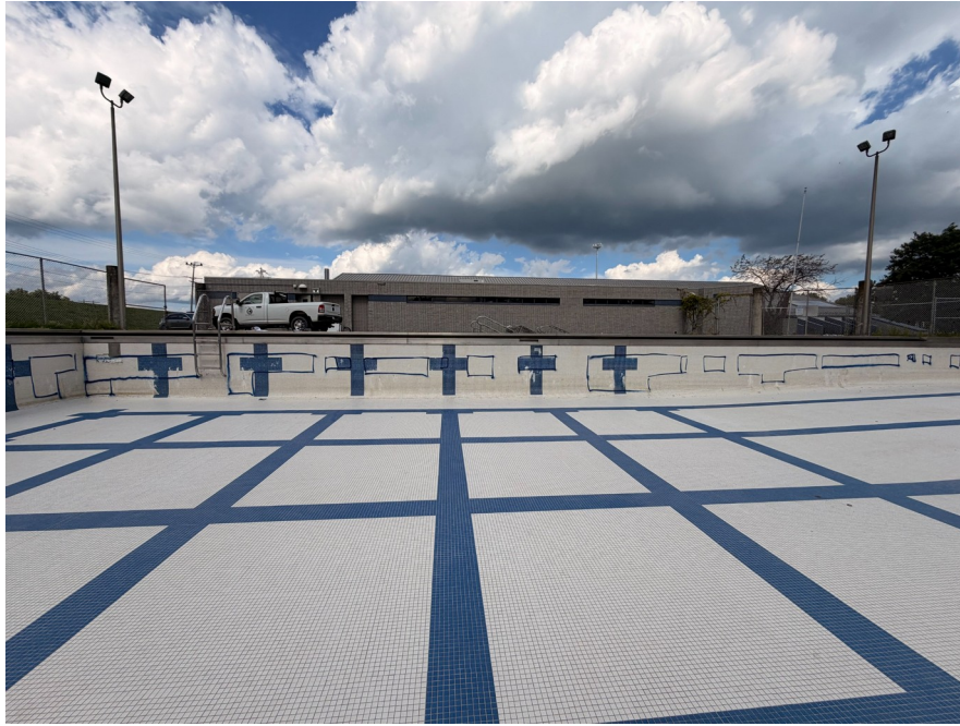
Photo 3 Wall facing the recreation center building. Blue-painted outlines document the areas identified during sounding.
