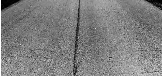
Centerline crack (still tight). ▶
