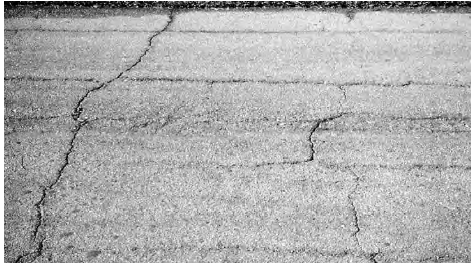
▼ Block cracking with open cracks.
