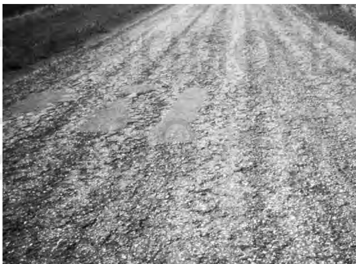
◀ Severe raveling and loss of surface material.
