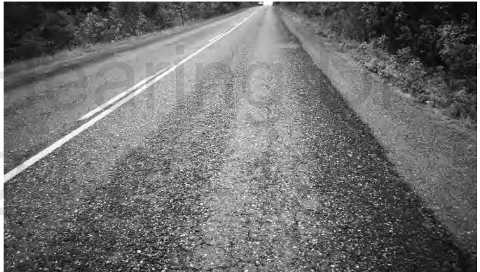
► Moderate to severe raveling in wheel paths.
