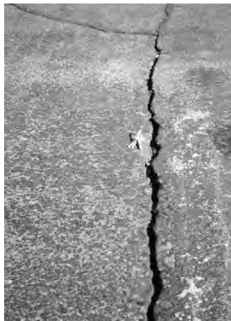
▲ Open crack – 1/2" or more in width.
