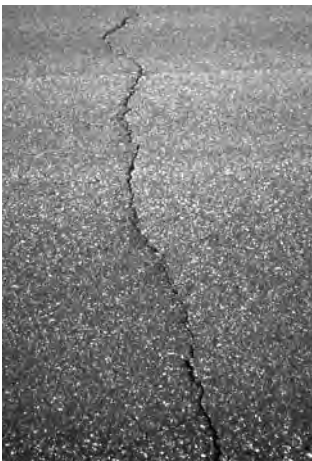
▲ Tight cracks less than 1/4" in width.
