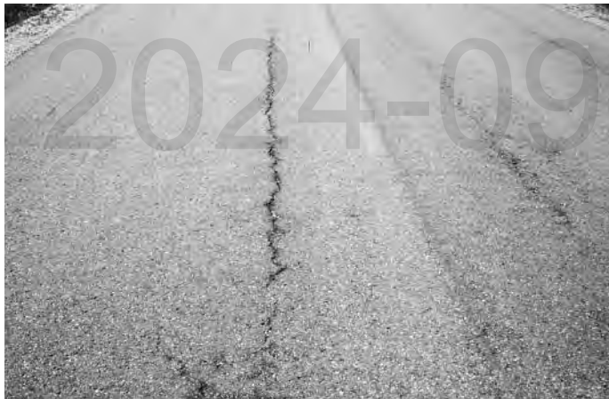
Multiple open, longitudinal cracks that are raveling. ▼
