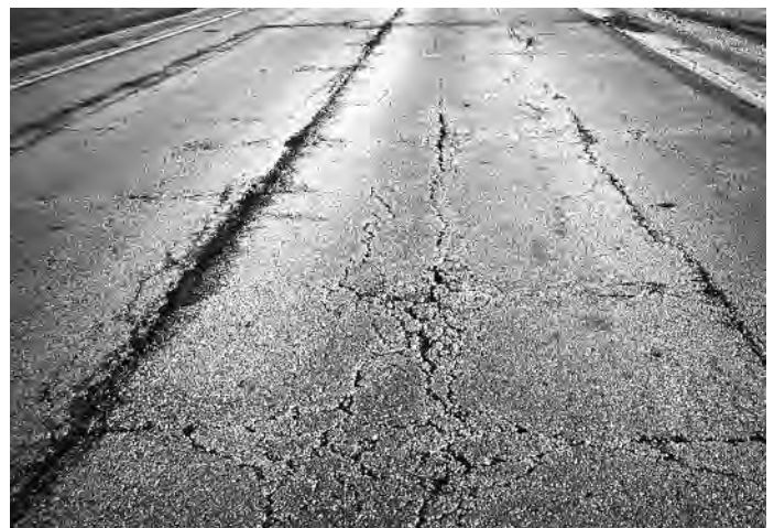
Multiple open, longitudinal cracks that are raveling. ▼
