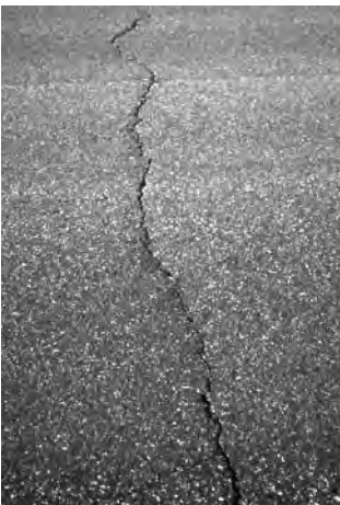
▲ Tight cracks less than 1/4" in width.
