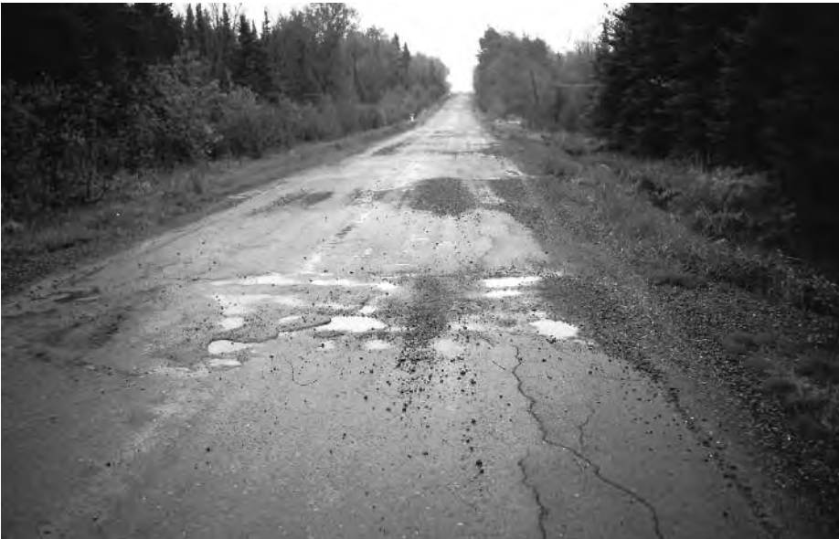
◀ Multiple potholes show pavement failure, probably due to poor subgrade soils, frost heave, and bad drainage.
