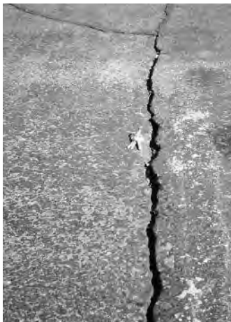
▲ Open crack – 1/2" or more in width.
