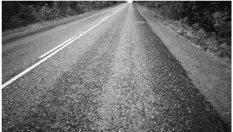
► Moderate to severe raveling in wheel paths.
