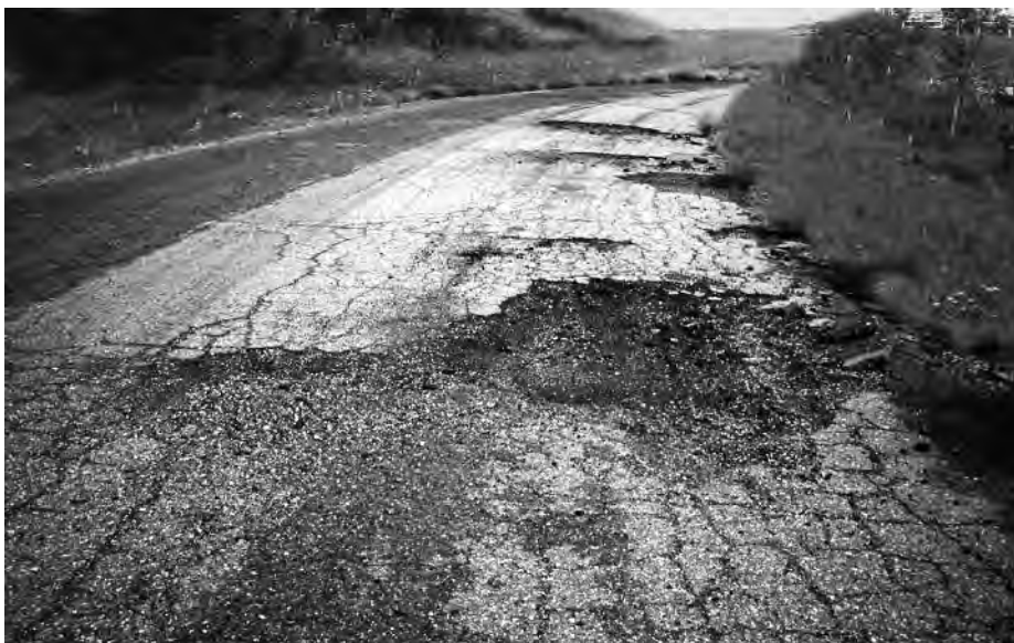
◀ Large, isolated potholes extend through base. Note adjacent alligator cracks which commonly deteriorate into potholes.
