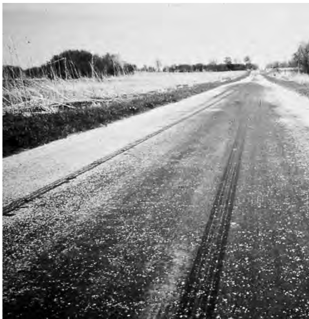
▼ Severe flushing.
