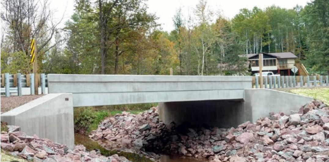
**Example Slab-Span Bridge**
