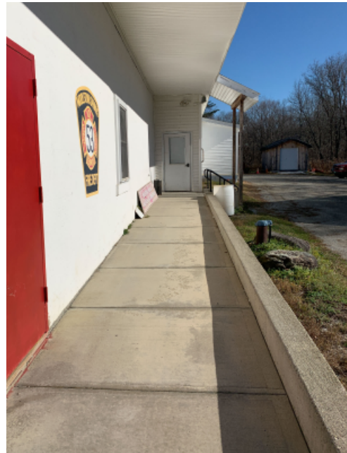
RAMP : The entrance ramp is not accessible. The ramp requires an accessible rail along the path of travel. The ramp itself is required to have rails at the side of the ramp. A intermediate landing is required at 12' of run. The rails at the stairs are not to code. The railing returns at the top and bottom run are not to code.
