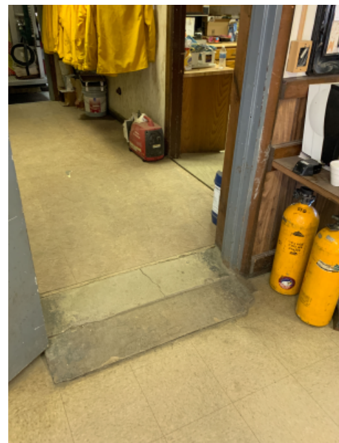
ROOM ENTRANCE : The middle portion of the 1950's section is raised from the apparatus bays. The raised floor is to allow for a crawlspace piping chase. The result however is that not all rooms are accessible, including storage rooms, kitchen, apparatus bays, and stage. This raised portion needs to be removed and all floors are to be on the same plane.
