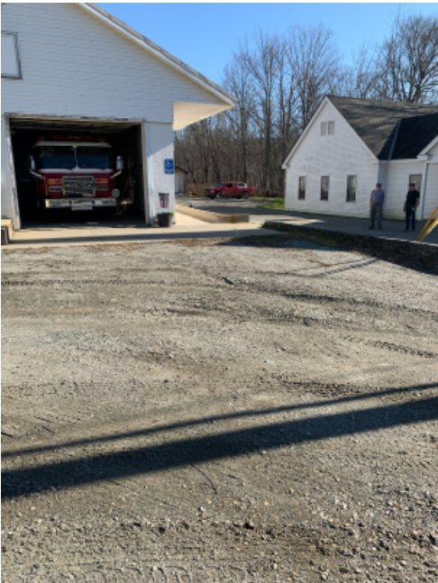
ACCESSIBLE BUILDING ACCESS: In order for a building to be accessible, designated accessible parking is required, near the building. An accessible pathway is then required to the main accessible entrance. Both elements are missing and are required.
