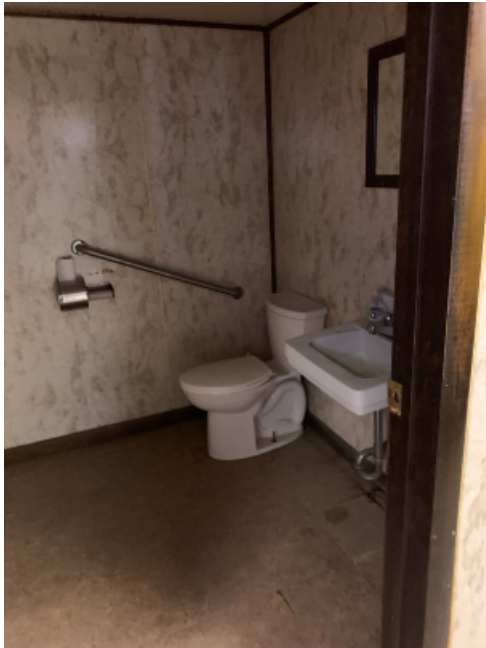
RESTROOM: The bathroom is not accessible. The plumbing fixtures are not accessible. The toilet grab bars are missing, and the one that is present is not to code. An additional bar is required. The existing bar is to be replaced and set at the correct height. The faucet levers are not to code, and need to be replaced with levers. The mirror is not to code, and needs to be replaced. Under counter piping insulation is required.
