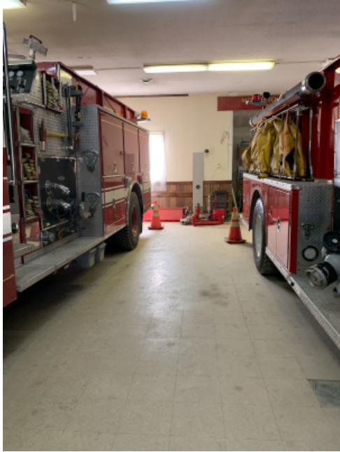
TRUCK SIZE VERSUS APPARATUS BAY SIZE: The fleet of fire trucks do not fit into the apparatus bay. The bay shown in this photo was designed as a bingo parlor and not as a garage. The trucks height barely fit the facility. The facility floor is vinyl tile and not a proper bay surface. No floor drain is present. Snow and water from trucks accumulates on the floor, creating a moisture and cleanliness issue.
