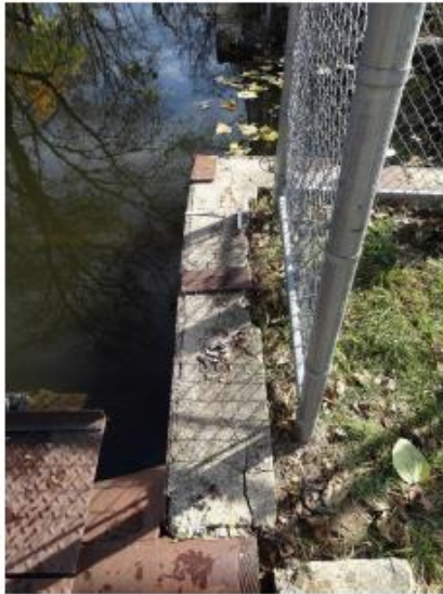
Photo 1 – Above: View of Benchmark 496-C, prior to demolition of dam. Spillway is to the left, under the steel plate; disk is to the right of the corner of the wall (cut off by edge of photo).
