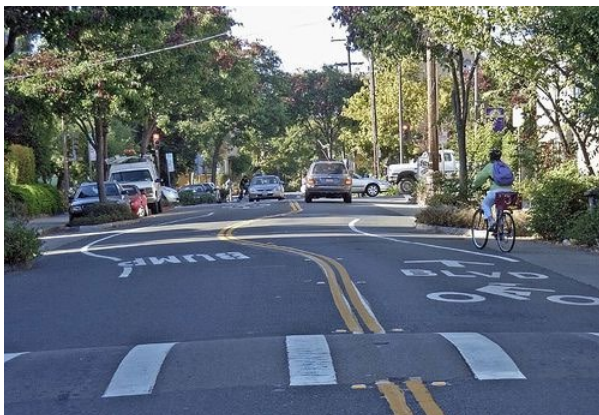
Figure 3-11: Bike route with chicanes to slow traffic flow. Source: Urban Street Design Guide, NACTO.
