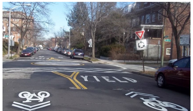
Figure 3-12: Mini roundabout with mountable apron and island that larger vehicles can drive over to negotiate turn. Source: Urban Street Design Guide, National Association of City Transportation Officials (NACTO).
