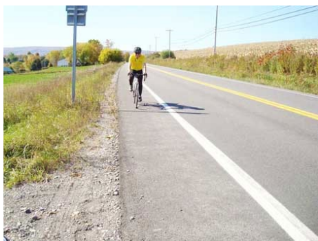
Figure 3-13: Paved shoulder. Source: Cornell Local Roads Program.
