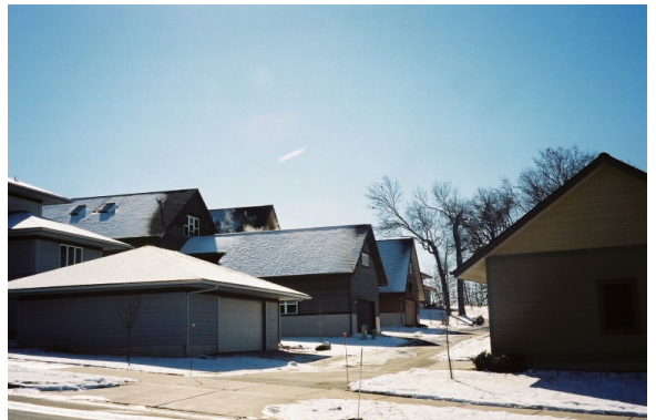
Figure 2-5: Alley for garages and rear lot access. Middleton Hills, WI. Source: Brown County Planning Commission.
