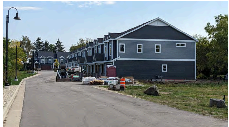
Figure 4-1 New Housing Construction
