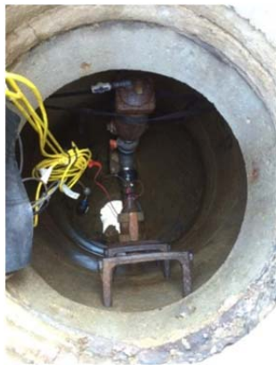
Figure #5: Air Relief Manhole
