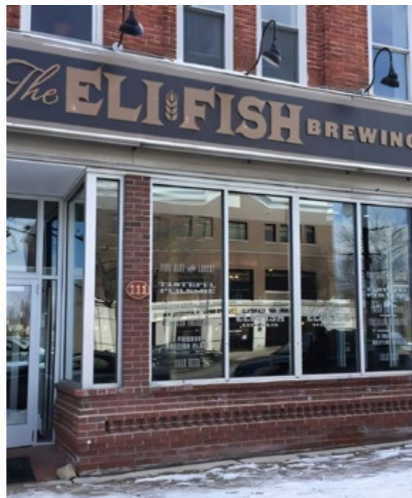
Example of a Completed Brewery Project (Batavia DRI Round 2)
