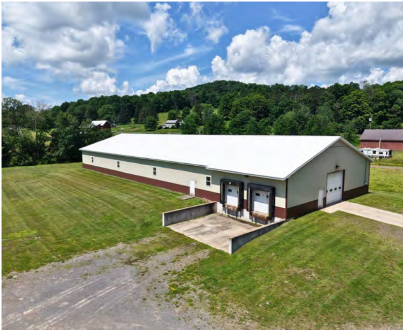
Existing Conditions at 5 Grant Pl
