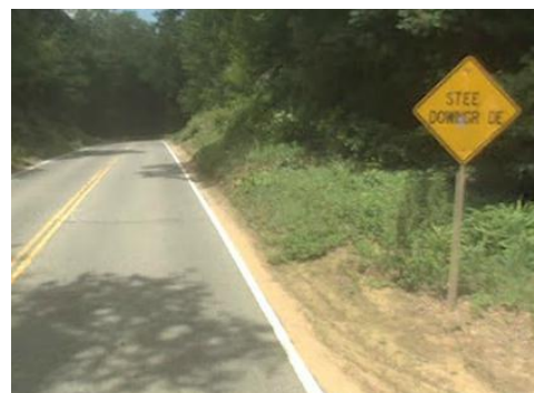
Substandard existing sign
