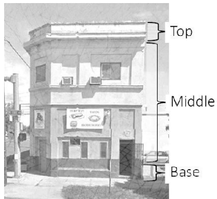
Figure 2.2.160B(3) –Building Base, Middle and Top
