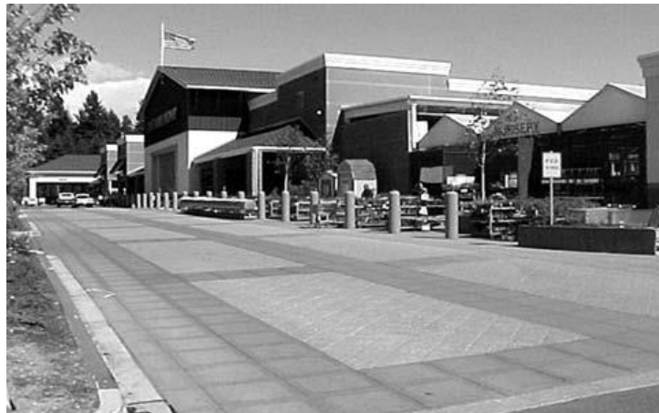
FIGURE 8-4C-7 DISTINCTIVE TEXTURE PATTERN ON PEDESTRIAN WALKWAY FLUSH WITH DRIVEWAY EXAMPLE
