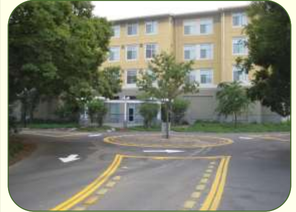
High volume intersections of two pathways may require special design features, such as this multi-use trail roundabout in Davis, CA.
