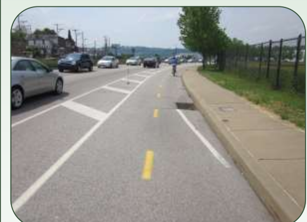
Drainage grates may also be marked with a diagonal line in the direction of travel so trail users can maneuver around them.
