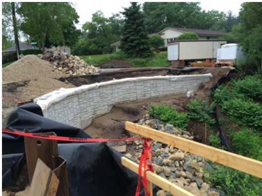
Concrete work is the main focus of project work. The new inlet structure is being constructed and reconnected to the seawall on the east side of the inlet structure. Once the new inlet structure is finished and the seawall is reconnected, the water will then be re-diverted to flow through the new spillway culvert structure.
