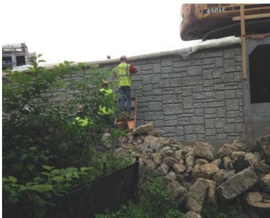
The decorative facing on the north permanent sheet pile wall has been constructed, except in the area of the diversion channel.
