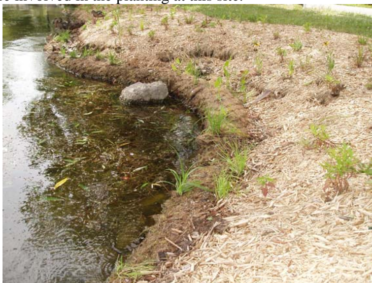
The fiber roll along the waters edge holds the shoreline in place while the new plantings get established on Pewaukee Lake.
