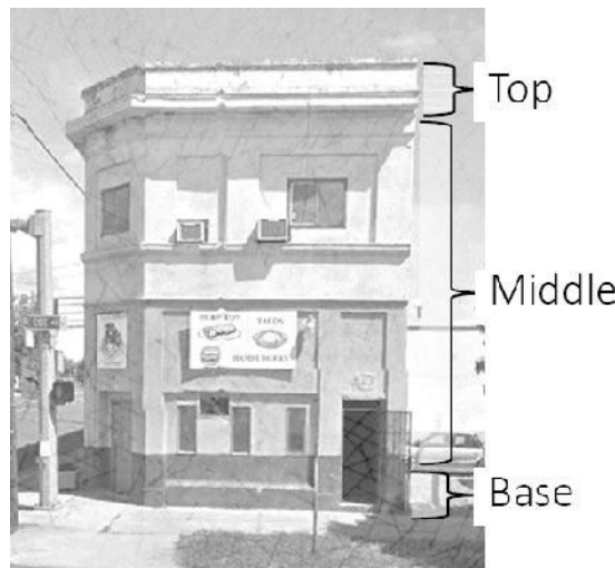
Figure 2.2.160.B(3) –Building Base, Middle and Top
