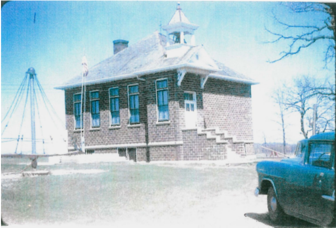
The historic school house in Nepeuskun, along with the other historic sites, is an example of the strong agrarian history of the town.
