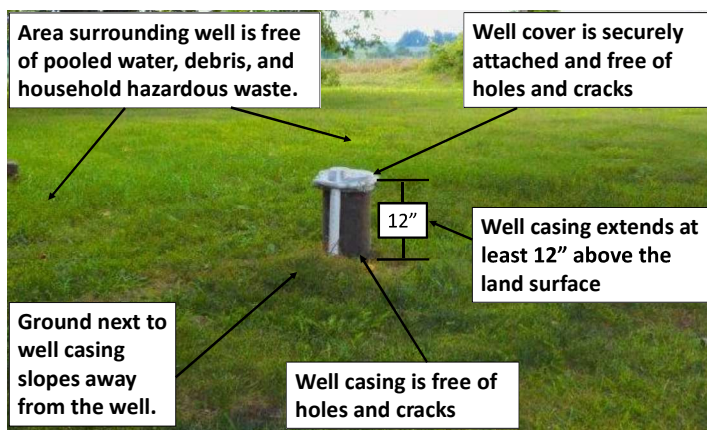
Figure 1: Photo of a properly constructed well.
