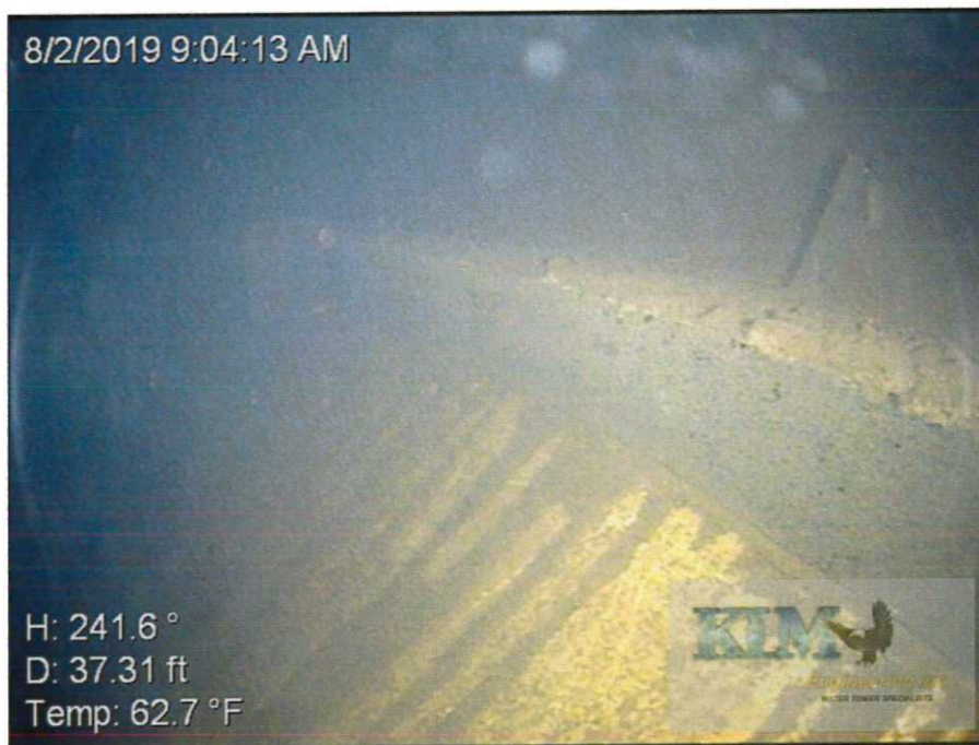
Photo No. 15 Condition of interior wet coating near tension ring Sediment accumulation and scale formation visible
