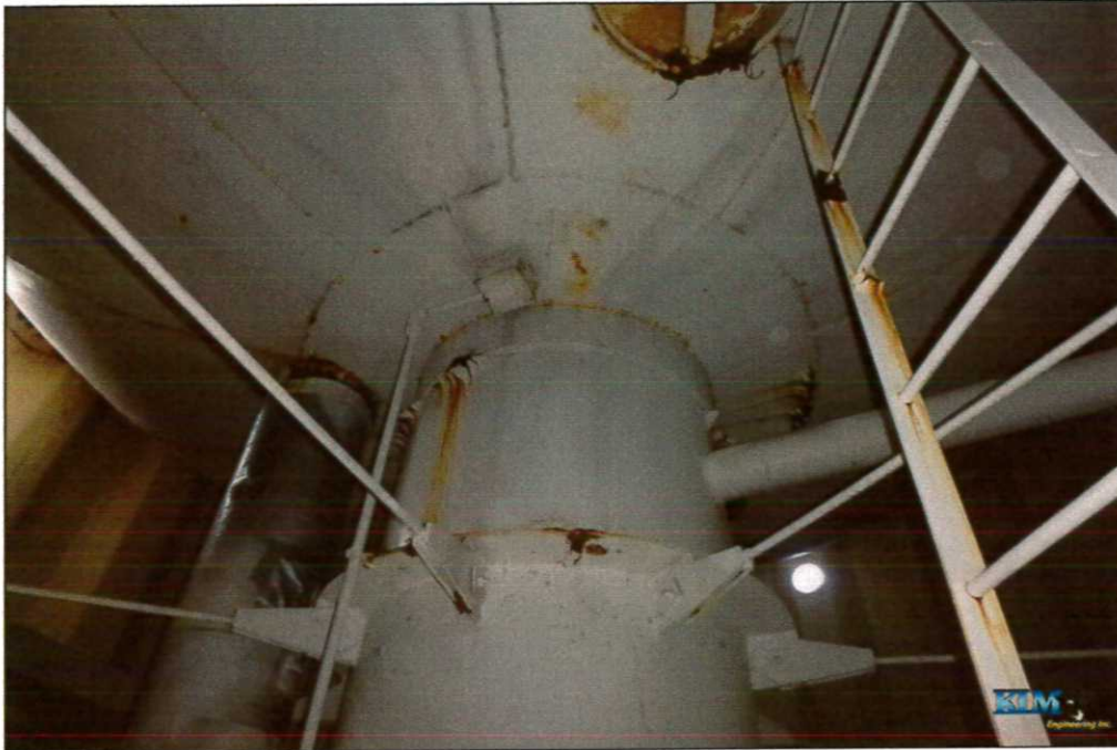
Photo No. 35 Overall condition of interior dry coating at bowl platform
