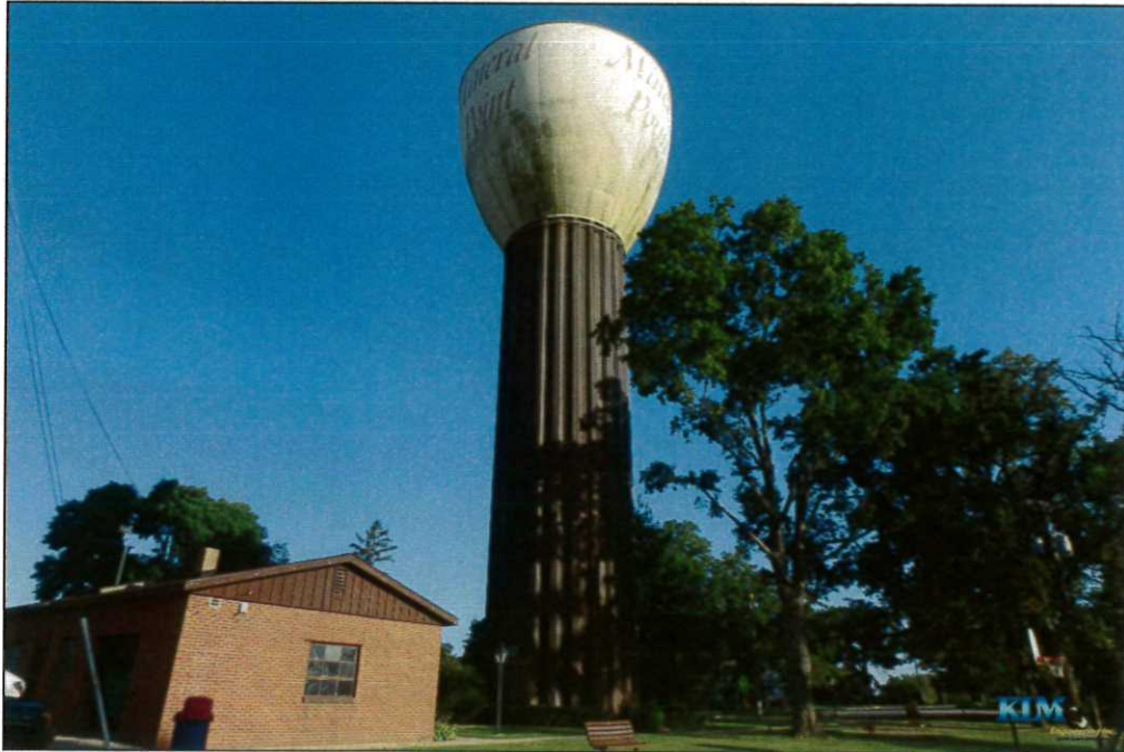
Photo No. 1 Overall view of tower
