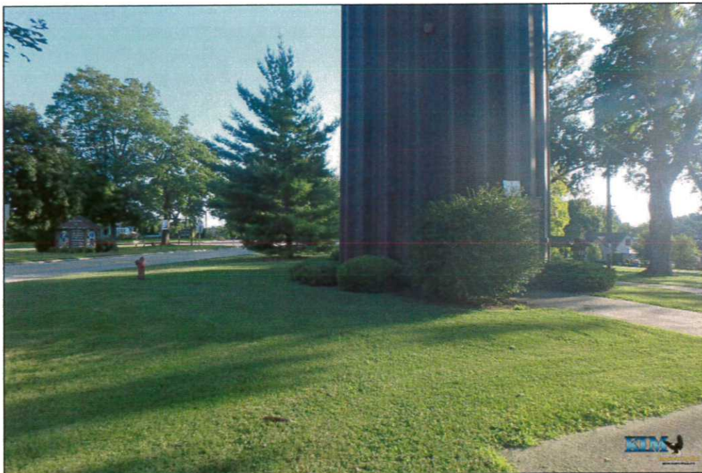
Photo No. 64 Site conditions near base of tower Hydrant for maintenance needs visible
