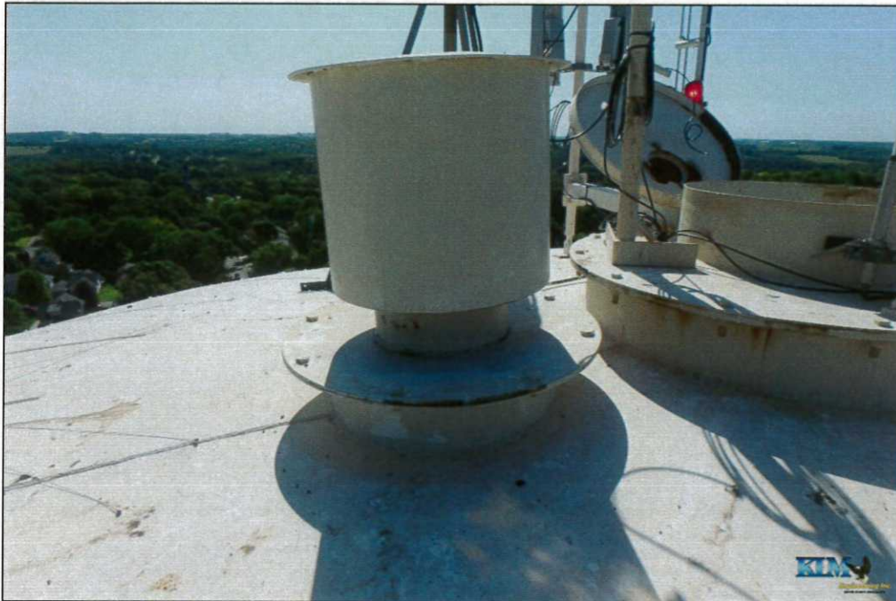
Photo No. 53 Condition of existing tank vent
