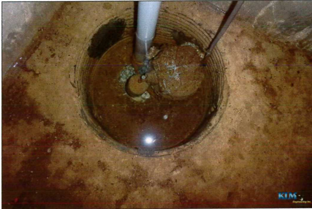
Photo No. 51 Condition of sump pump in valve pit
