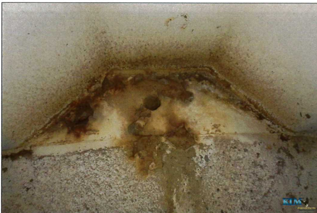
Photo No. 42 Condition of condensate platform drain-pipe connection
