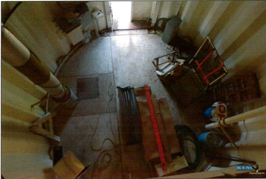
Photo No. 43 Overall view of conditions inside base of pedestal
