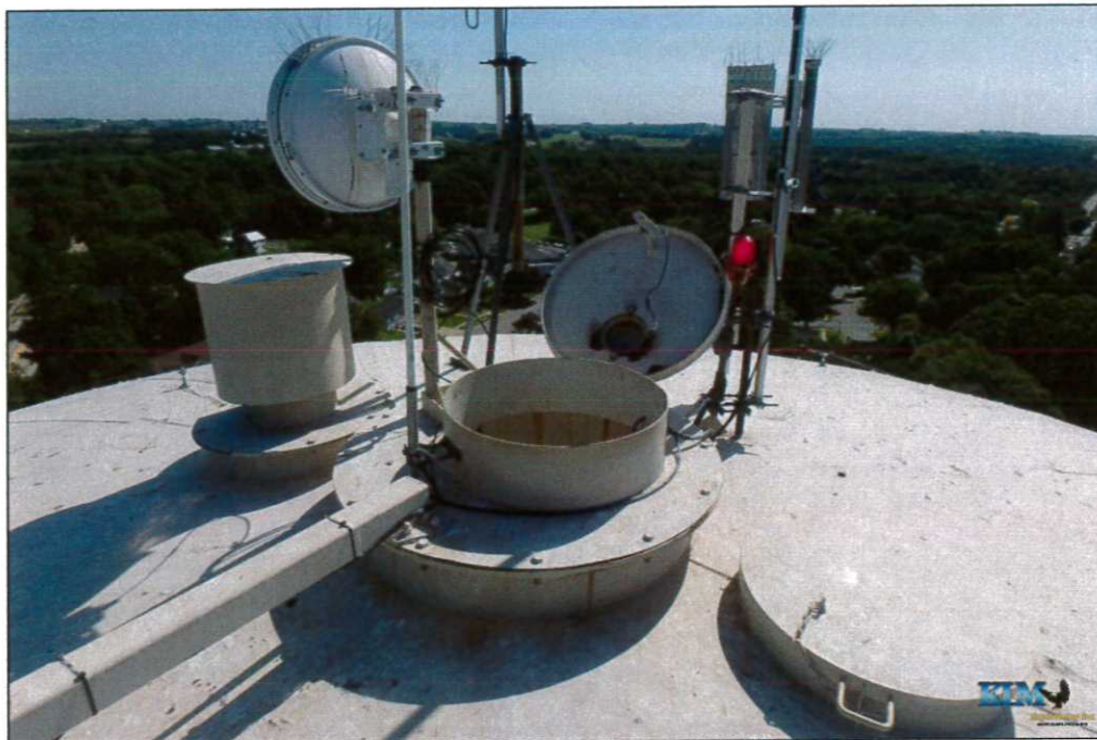
Photo No. 52 Overall view exterior roof condition
