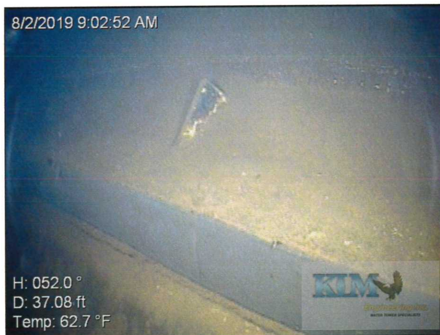
Photo No. 16 Condition of interior wet coating near tension ring Heavy sediment accumulation visible
