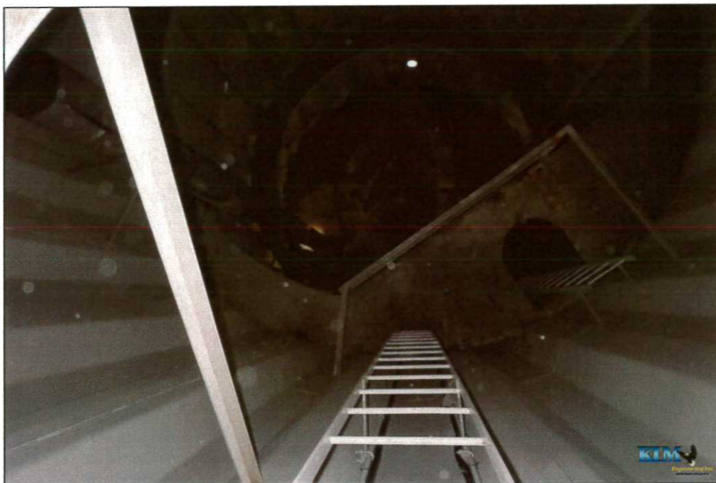
Photo No. 40 Condition of access ladders and wall coating inside pedestal
