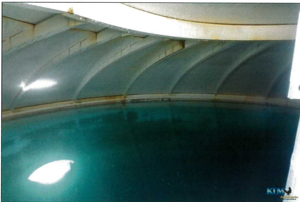
Photo No. 2 Overall condition of interior wet coating above HWL
