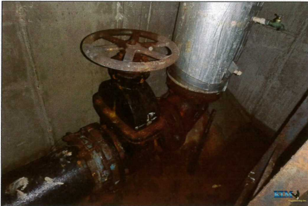
Photo No. 49 Condition of piping, valves, and fittings inside valve pit
