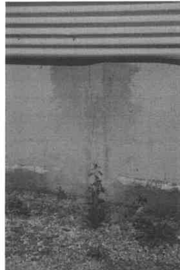
Previously Repaired Crack East Side Training Room Associated with Northeast Corner Settlement
