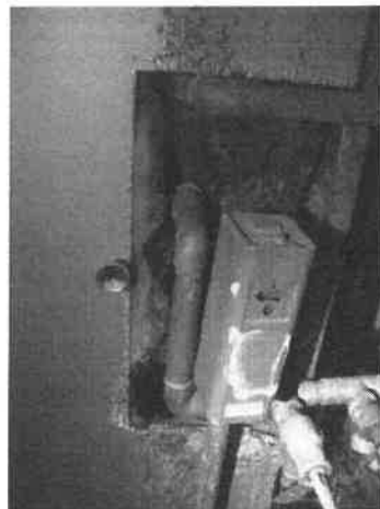
Observed rust at integral exchanger
