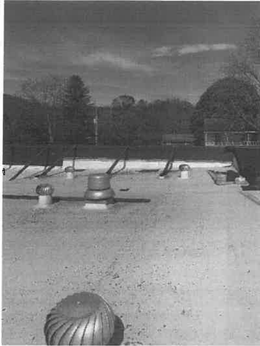
Membrane Roofing
