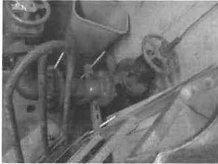
Domestic Cold Water Service Entry
