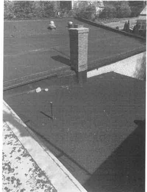
Membrane and Roll Roofing
