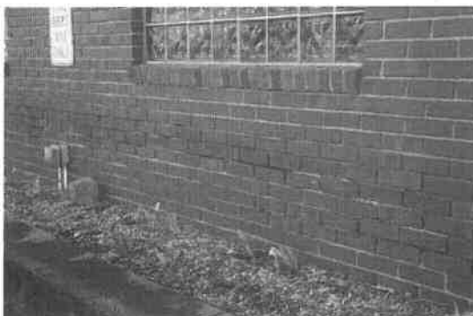
Mortar Joint Erosion West Wall Day Room
