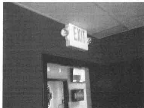
Figure 6 combination exit sign and ELU
