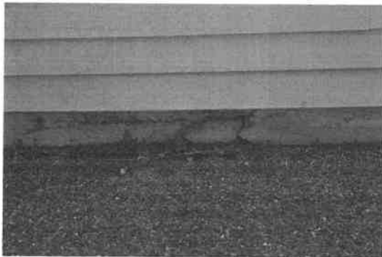
Foundation Crack South Side Apparatus Bays
