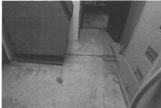
Crack in Floor Finish
