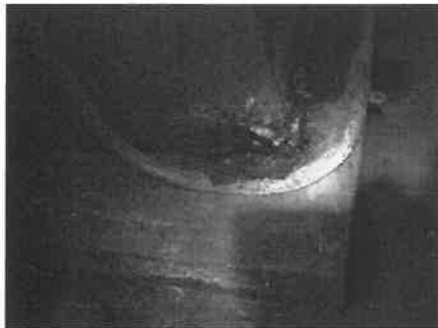
Observed rust at front boiler section
