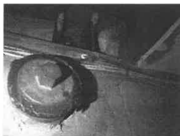
Figure 17 grounding electrode conductor
