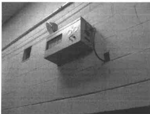
Figure 5 emergency lighting unit-ELU
