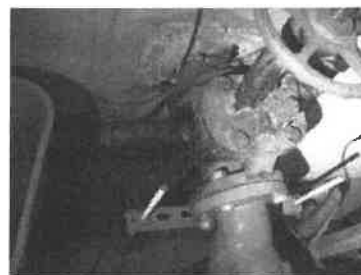
Figure 18 grounding electrode conductor
