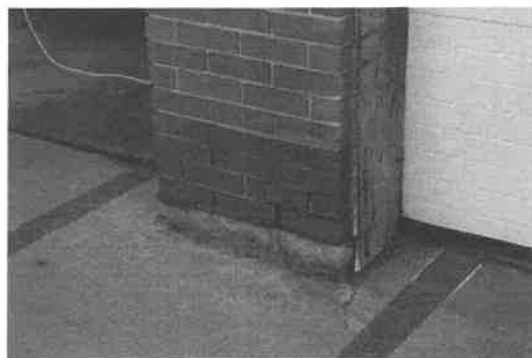
Mortar joint Erosion and Foundation Erosion West Wall Apparatus Rave
