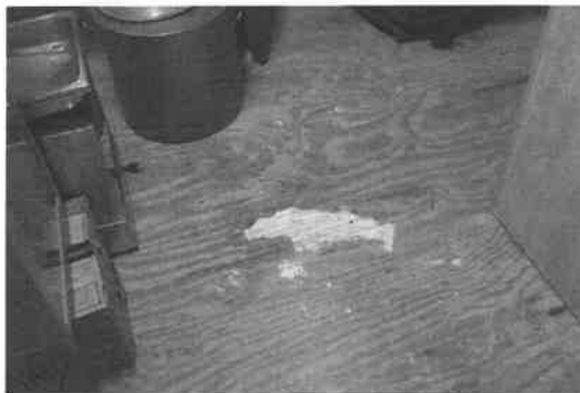
Water Damaged Floor Sheathing
