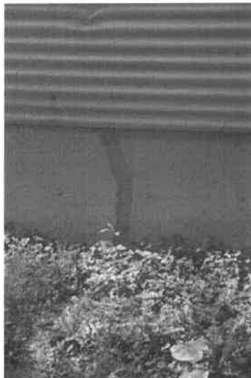
Previously Repaired Crack North Side Training Room Associated with Northeast Corner Settlement
