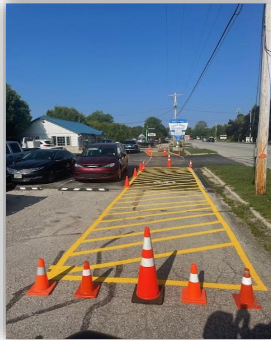
Striping on Hwy 42 trail
