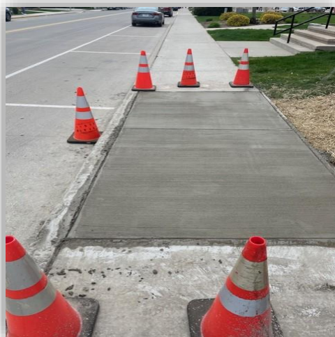
Concrete sidewalk by the Village Hall poured by the Parks/Maintenance employees
