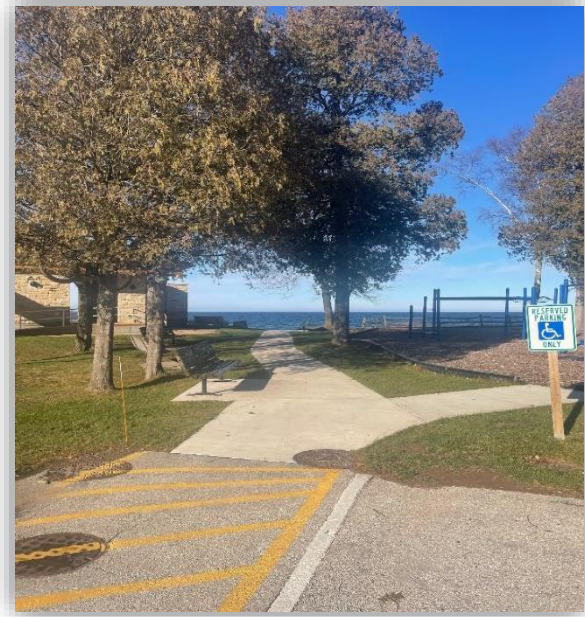
After the sidewalk was installed
