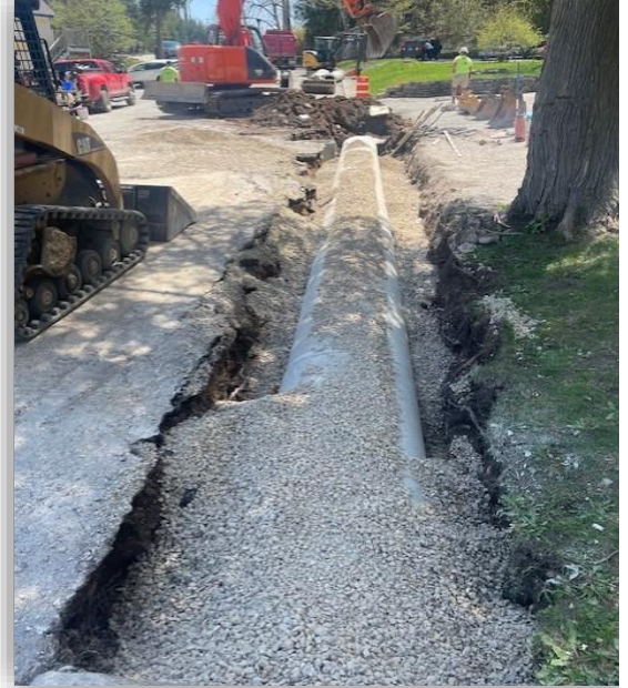
Bluffside Storm Sewer Replacement Project (After Repairs)
