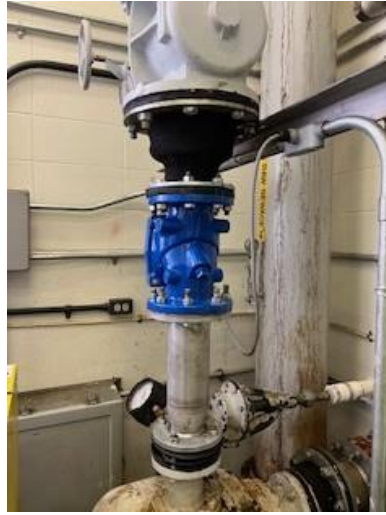
Picture 1.7 – New check valve that was installed on the main lift station pump #1.
