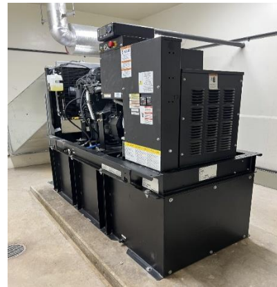
Picture 1.11 – New Little Sister Lift Station generator that was installed by Crane Engineering.
