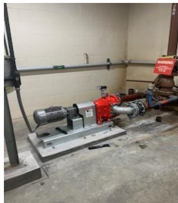
Picture 1.10 – New concentrated sludge pump that was installed by Crane Engineering.
