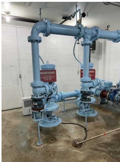
Picture 1.2 – The new check valves that were installed on the booster pumps at Well #2.
