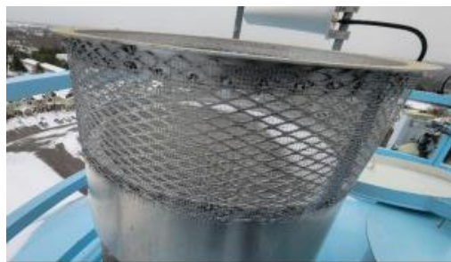
Picture 1.5 – The 4-mesh vent screen that was installed on the Jungwirth Court water tower to meet DNR code requirements.
