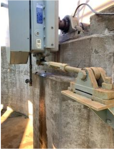
Picture 1.6 – Disc aerator drive that was leaking oil and was repaired.
