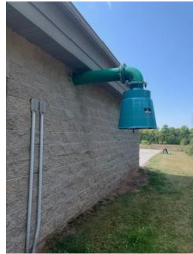
Picture 1.8 – New pretreatment blower intake filter and diffuser was installed.
