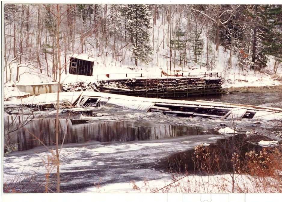
1994 storm surge damage – photo courtesy of Sharon Thompson (Orland Historical Society).
