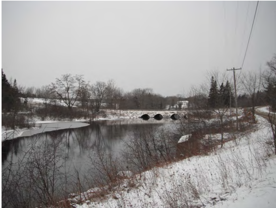
Upper Falls Road crossing from upstream.
