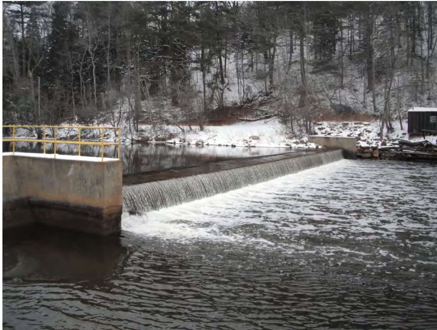
Dam spillway from downstream of right abutment. Note the high tide line on dam.
