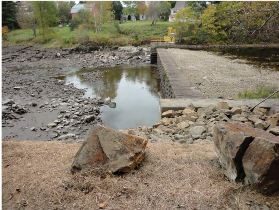
Dam from left abutment following 2012 repair work by Town.
