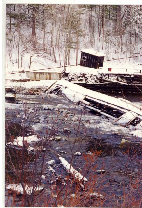
1994 storm surge damage – photo courtesy of Sharon Thompson (Orland Historical Society).
