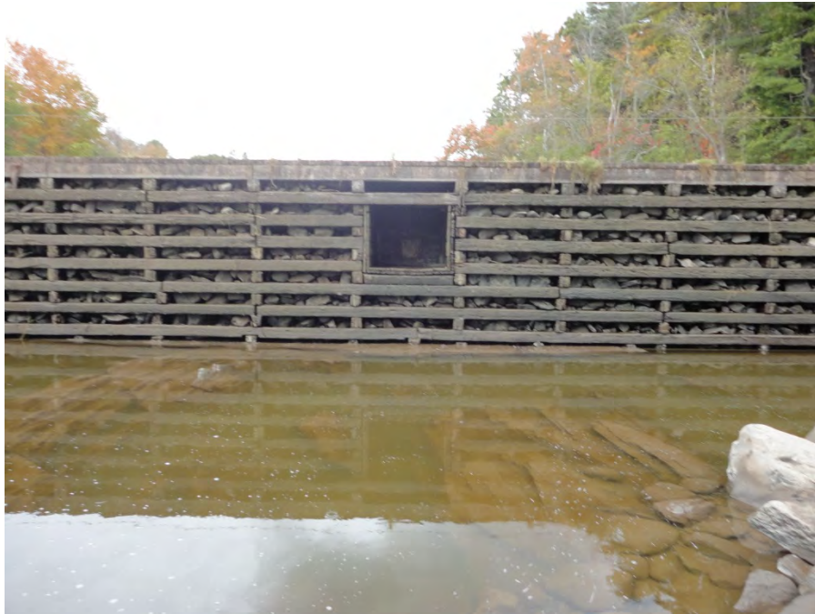
Timber crib section of dam.
