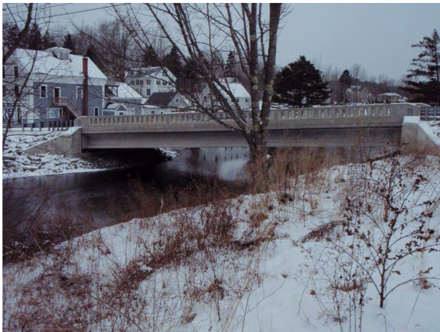
State Route 175 Bridge from downstream.
