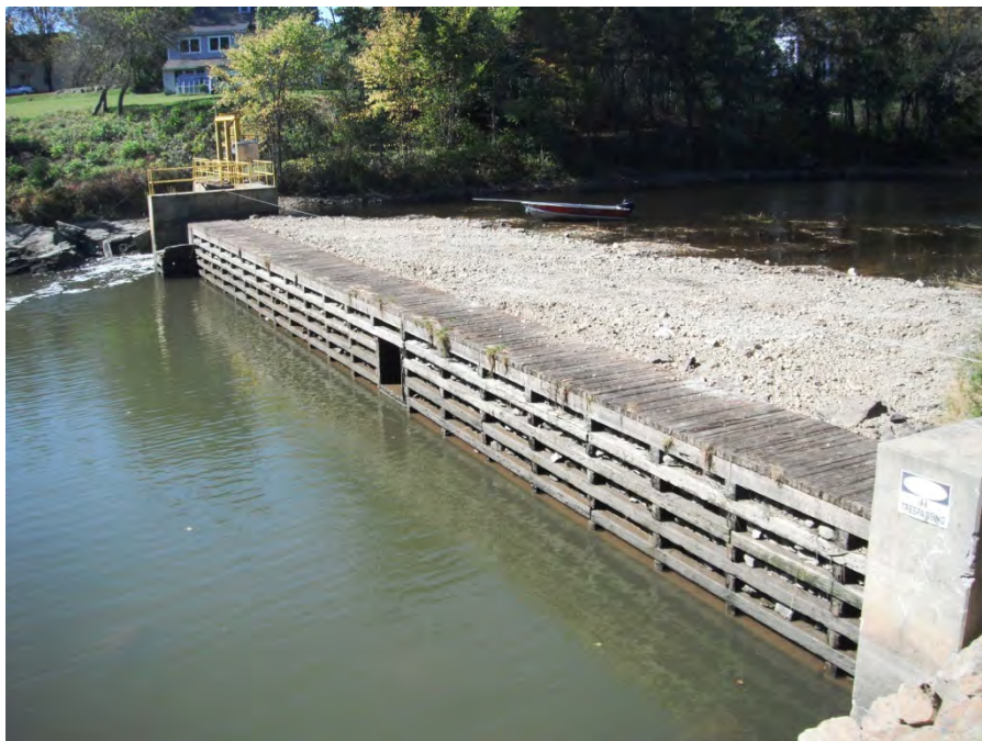
Dam following 2012 repair work performed by Town.
