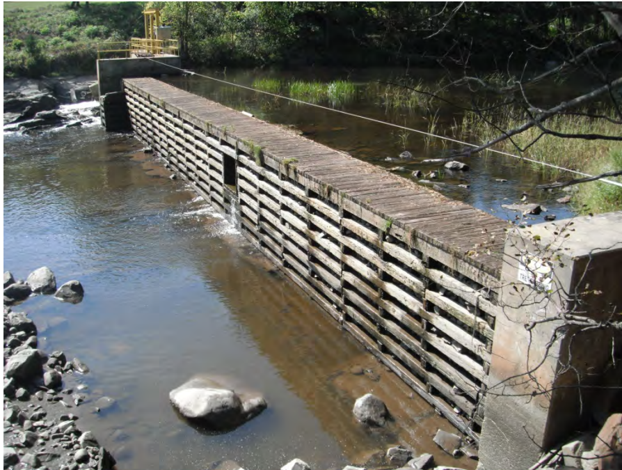
Dam prior to 2012 work performed by Town.
