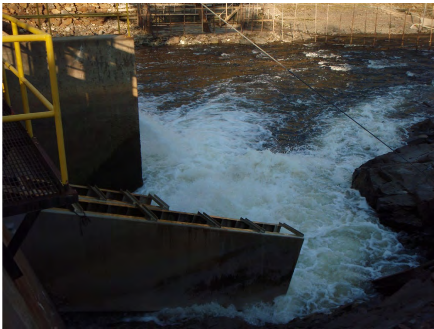
Fishway (operational, but non-functional) at low tide with flow over the dam. Note the alewife harvesting operations in background
