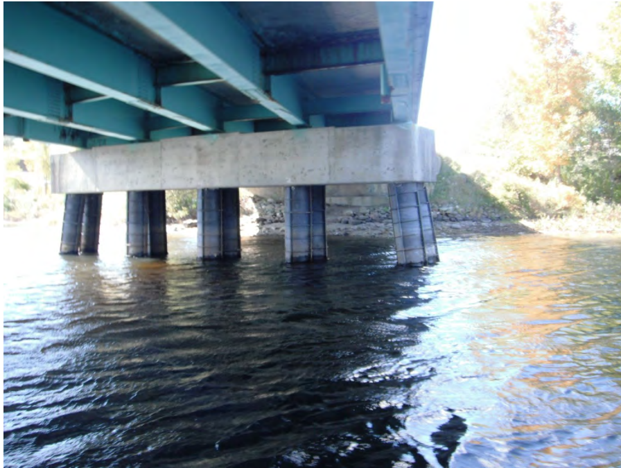
US Route 1 Bridge looking west.
