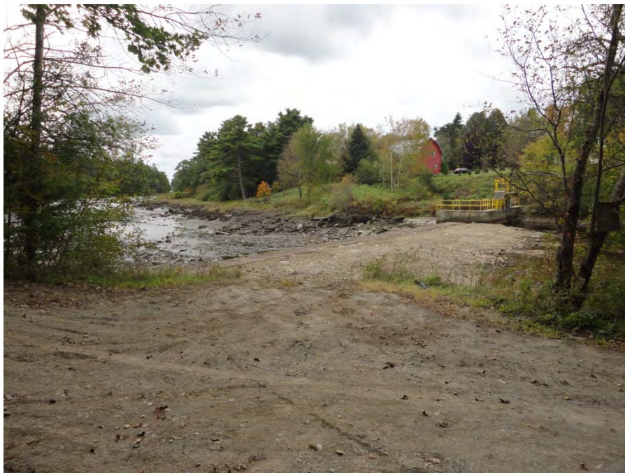
Dam from upstream of left abutment following 2012 repair work by Town.
