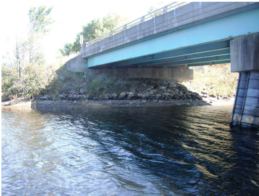
US Route 1 Bridge looking east.
