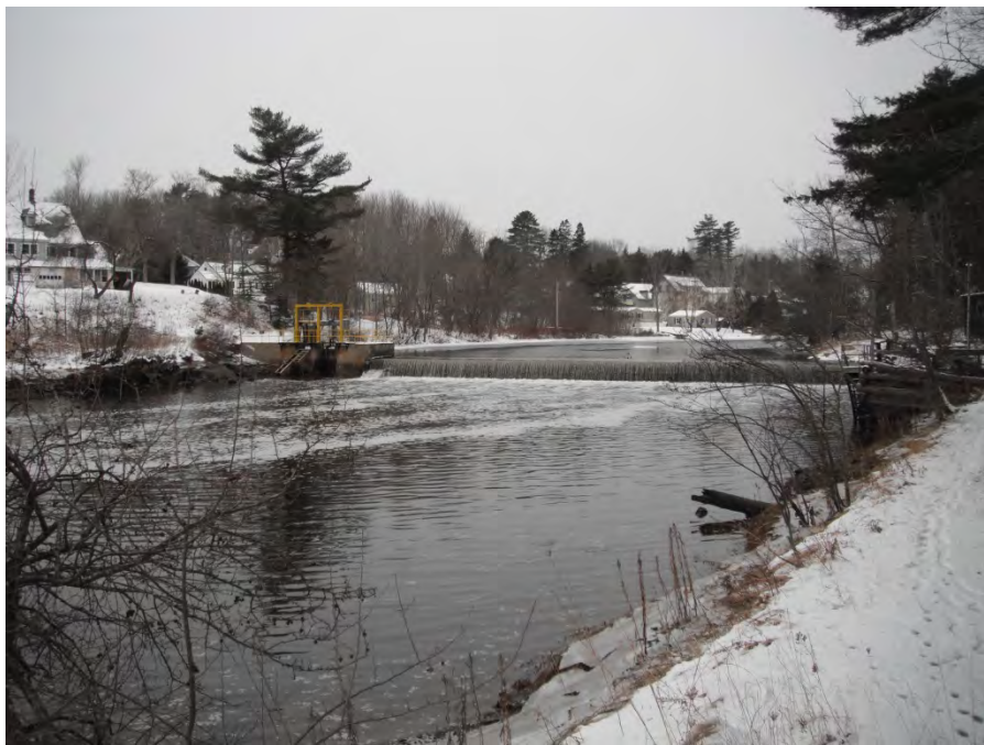
Dam from downstream of left abutment. Note the high tide line on dam.
