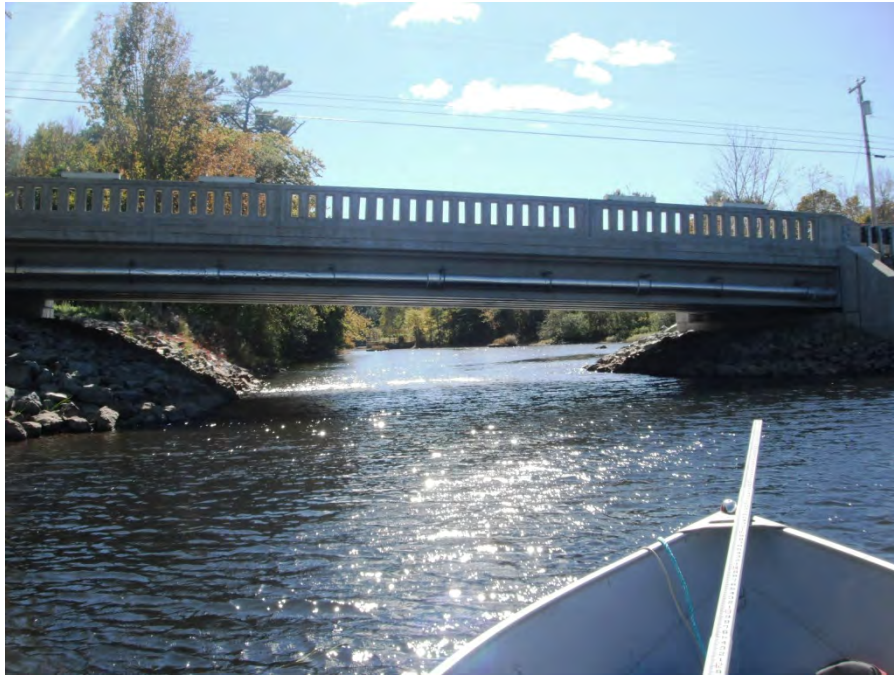
State Route 175 Bridge from upstream.
