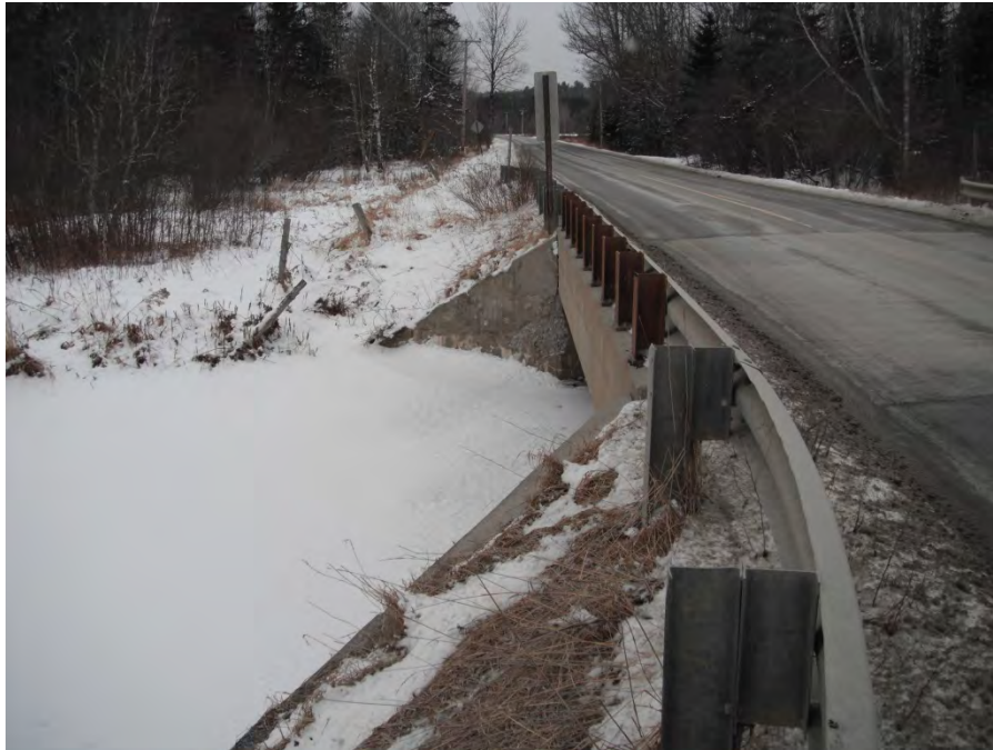
State Route 46 Bridge over White's Brook.
