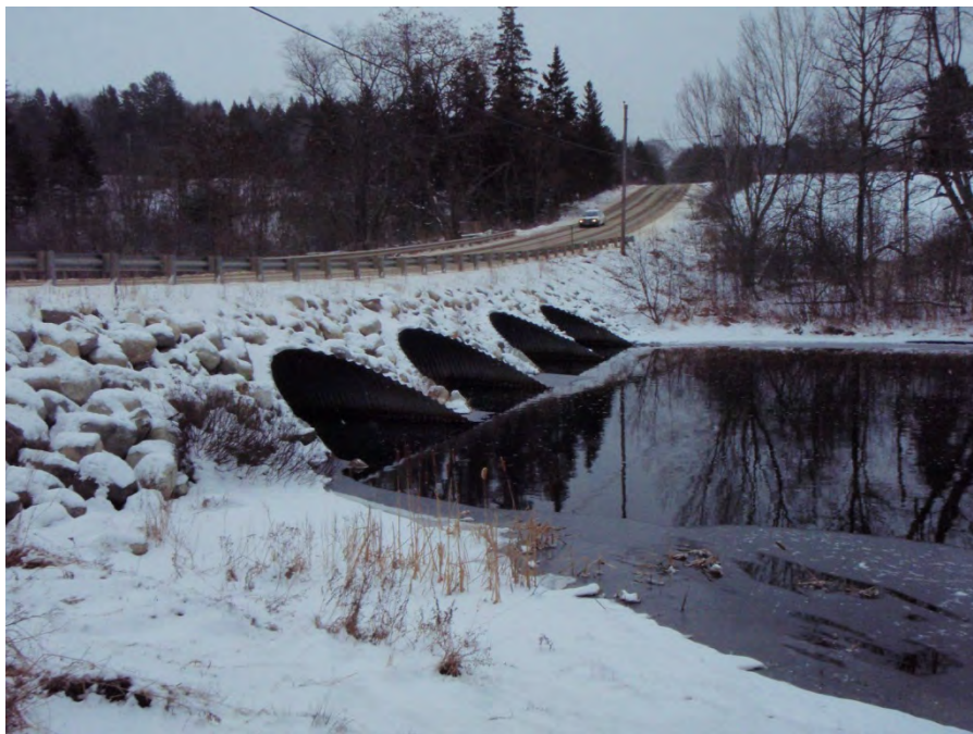
Upper Falls Road crossing from downstream.
