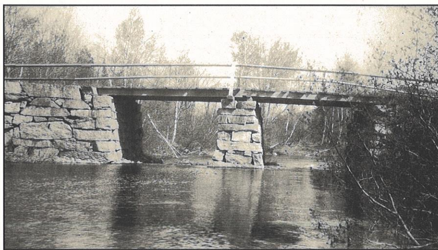
Moosehorn Creek bridge, near the Orland-Bucksport line, May 23, 1924.
