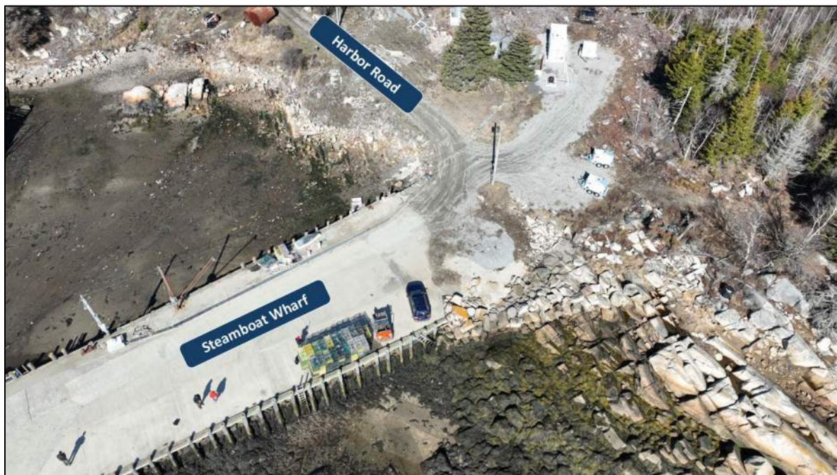
Figure 5-7. Aerial View of connection between Harbor Road and Steamboat Wharf
